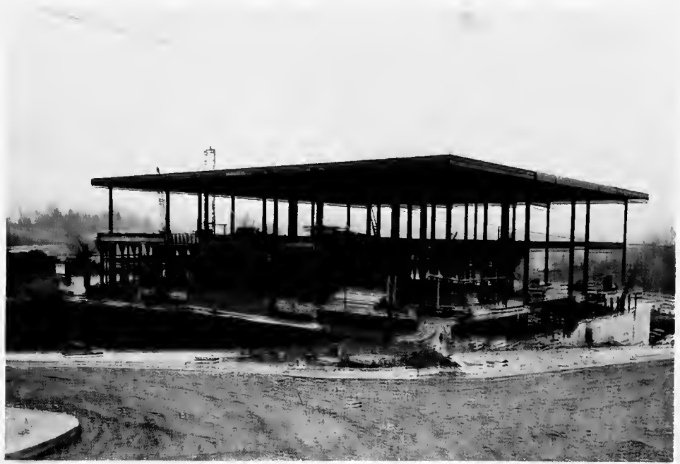
Classroom building under construction.
