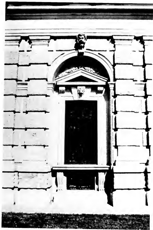
10. The wall and mask "dressed". Burgtheater, Vienna (Designed 1873 by Semper, executed by Hasenauer)
