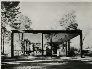
Glass House: Exterior (Photograph by Alexander Georges, from Kenneth Frampton, The Glass House Revisited, #52).
