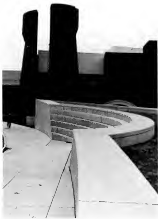
Wexner Center for the Visual Arts, Columbus, Ohio, Peter Eisenman with Dick Trott, Architects, Detail of Entry Court (Photograph by Ellen Stoner).
