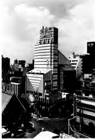
Niban-kan Building, Tokyo, 1970. Minoru Takeyama, architect (Photograph: Botond Bogner).
