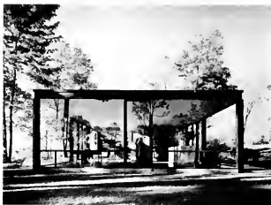
Glass House: Exterior (Photograph by Alexander Georges, from Kenneth Frampton, The Glass House Revisited, #52).
