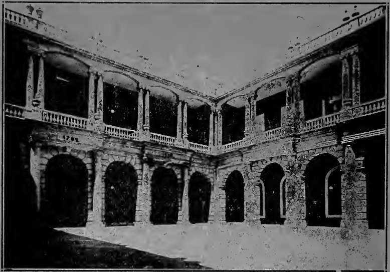
PATIO DE MINERIA. Inner Court in Mining School, Mexico City.
