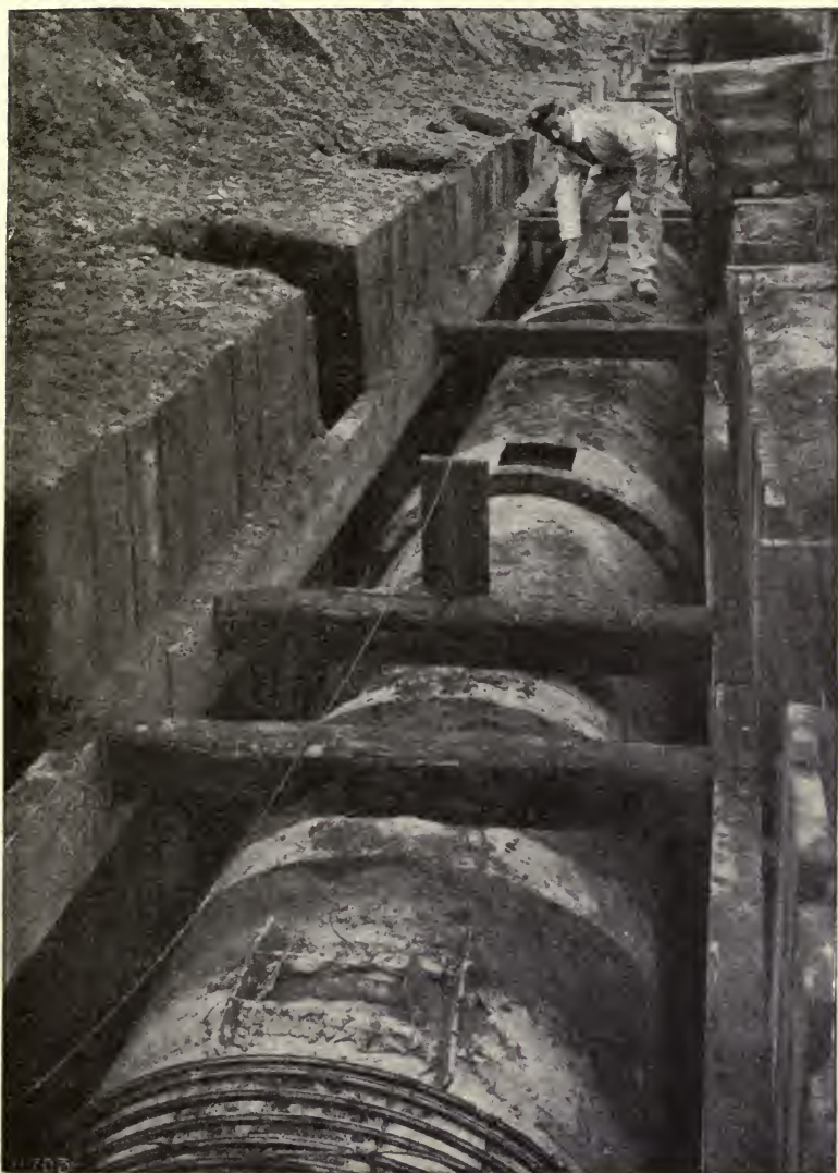
"Concrete and Constructional Engineering." FIG. 166.
