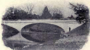
150' Span Melan Arch Bridge for F.W. Vanderbilt Rutledge Creek, Middleburg, Kentucky
