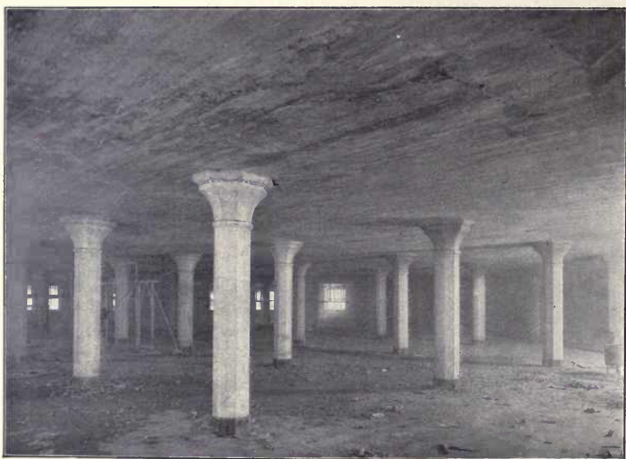
Fig. 124.—Interior of Bovey Building, Built by the Mushroom System. (See p. 190.)
