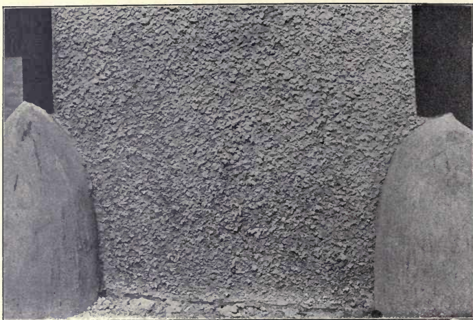
Fig. 129.—Photograph of Spatter Dash Finish of Lynn Storage Warehouse. (See p. 196.)
