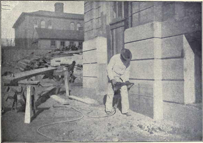
Fig. 127.—Tooling the Surface of Friedenwald Building Walls. (See p. 196.)
