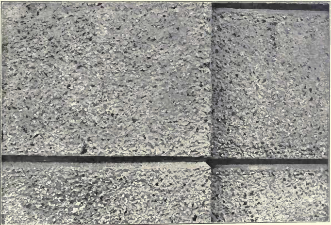
Fig. 128.—Photograph of Tooled Surface. (See p. 196.)
