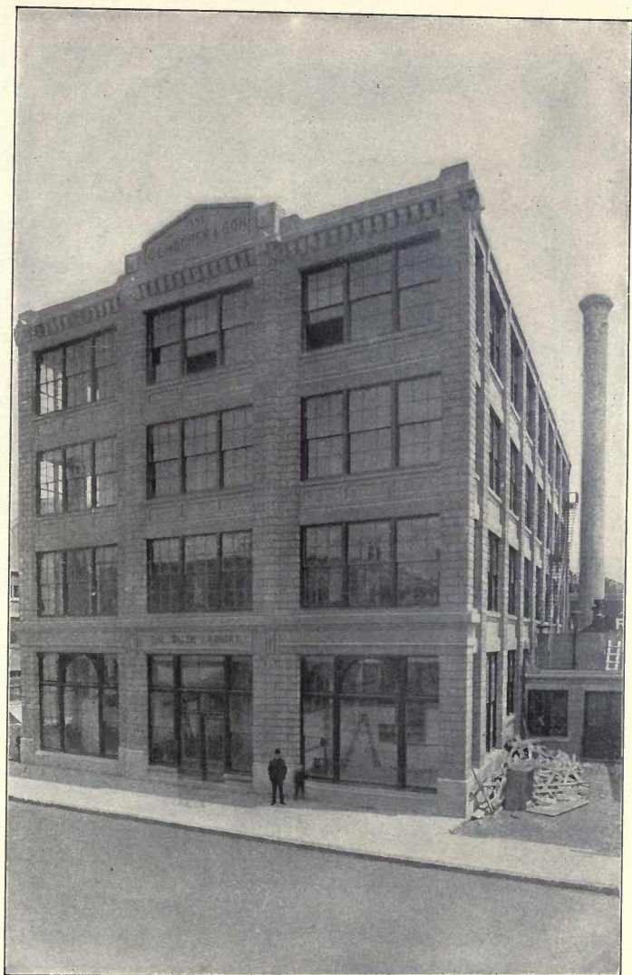
Fig. 125.—Concrete Block Walls, Salem Laundry. (See p. 195.)
