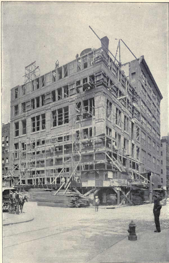
Fig. 22.—Exterior of the Ketterlinus Building During Construction. (See p. 69.)
