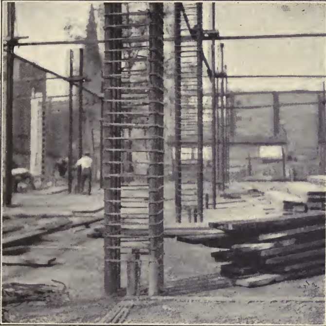
FIGURE 82. COLUMN REINFORCEMENT
