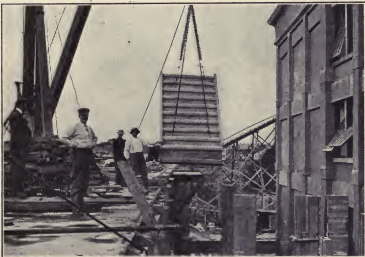
FIGURE 140. SETTING A FLIGHT OF STAIRS.
