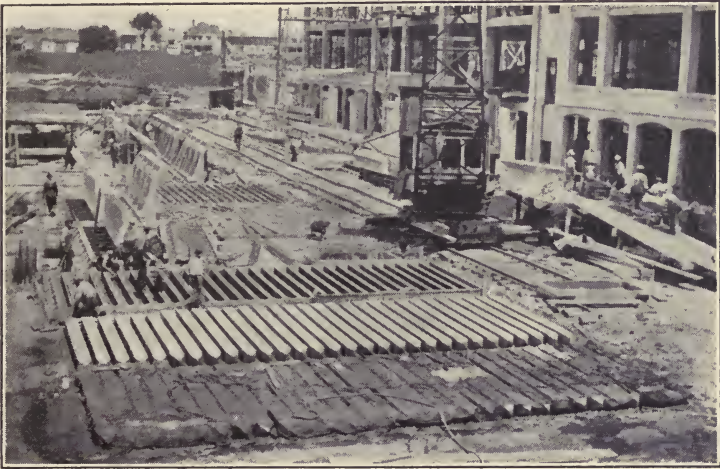
FIGURE 143. MANUFACTURING REINFORCED CONCRETE PILES.
