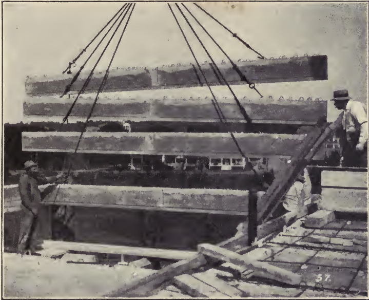
FIGURE 139. SETTING THE BEAMS.
