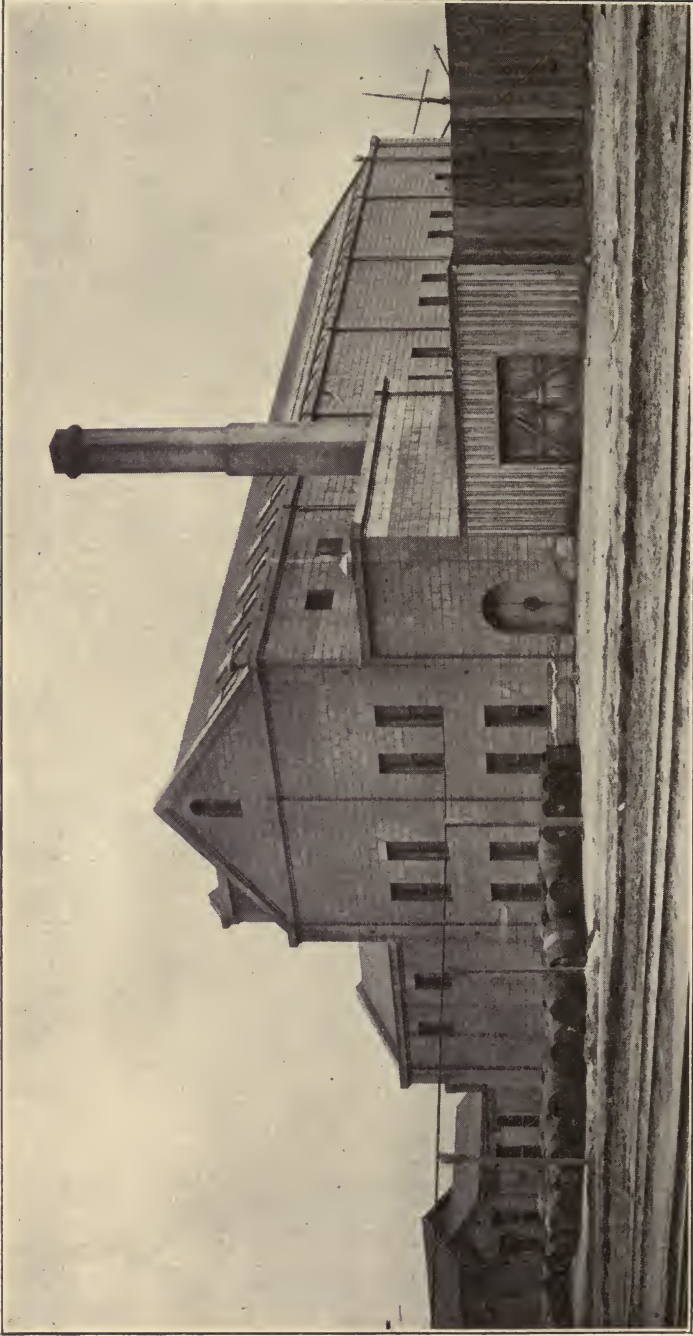
ARCTIC OIL WORKS, SAN FRANCISCO Reinforced Concrete Walls and Columns; erected by Ernest L. Ransome, 1884
