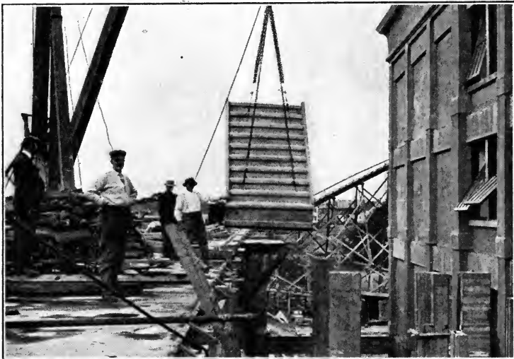
FIGURE 140. SETTING A FLIGHT OF STAIRS.
