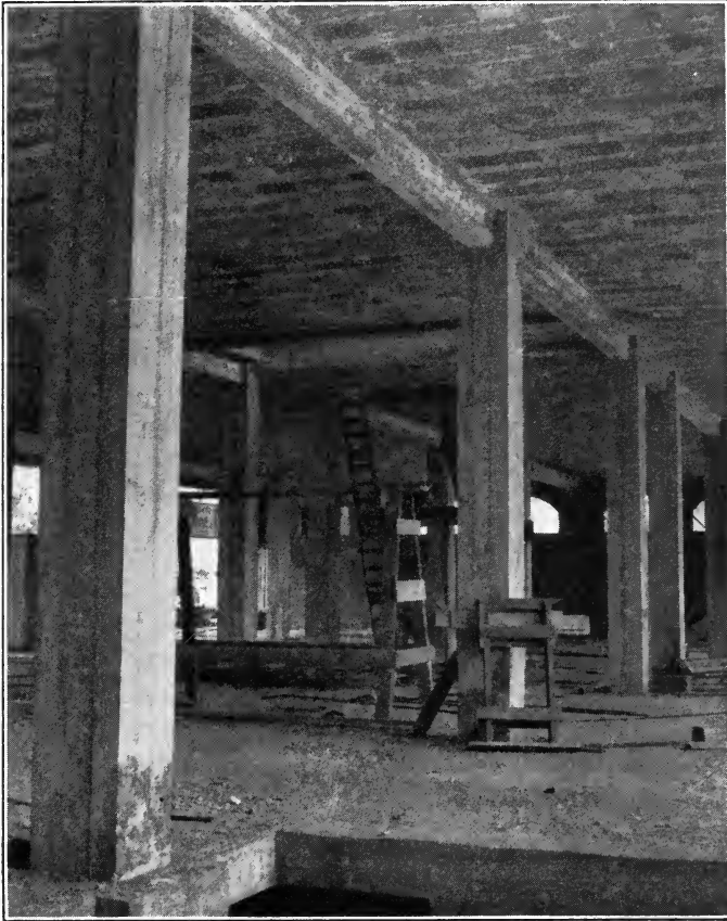
FIGURE 89. TILE CONCRETE CONSTRUCTION, READY FOR PLASTERER
