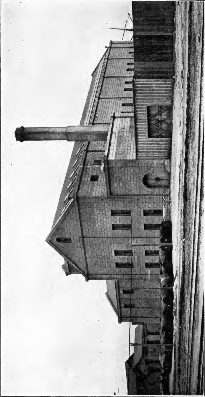
ARCTIC OIL WORKS, SAN FRANCISCO Reinforced Concrete Walls and Chimney; erected by Ernest L. Ransome, 1884
