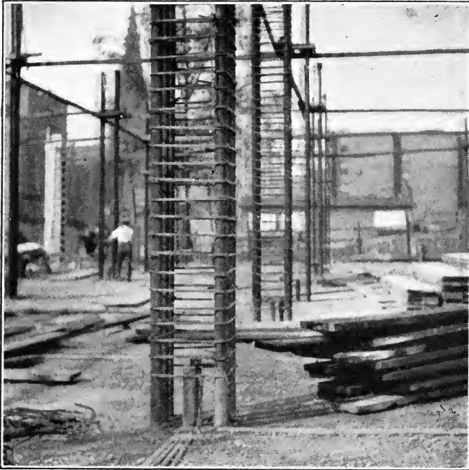
FIGURE 82. COLUMN REINFORCEMENT
