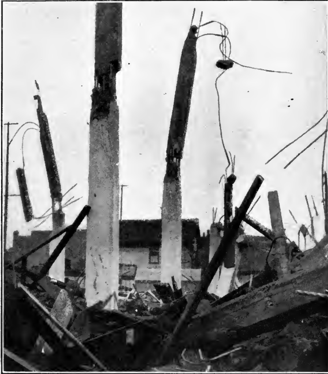
FIGURE 147. WRECK OF THE HENKE BUILDING IN CLEVELAND.
