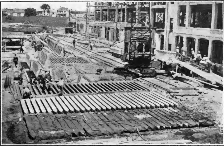
FIGURE 143. MANUFACTURING REINFORCED CONCRETE PILES.
