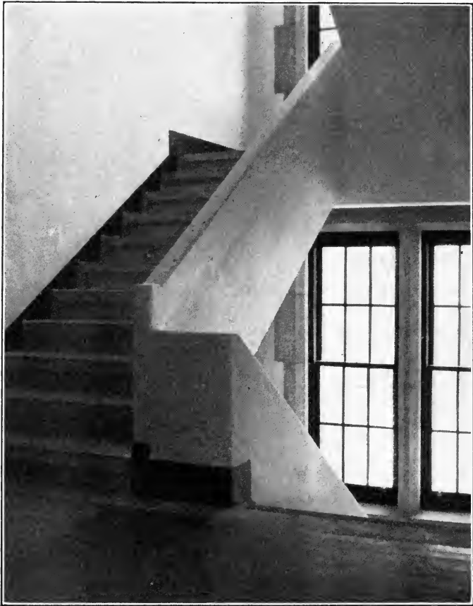
FIGURE 145. MONOLITHIC CONCRETE STAIRS AND RAIL, CAST IN ONE PIECE THREE STORIES HIGH. CONCRETE WAS RUBBED WITH CARBORUNDUM AND PAINTED.
