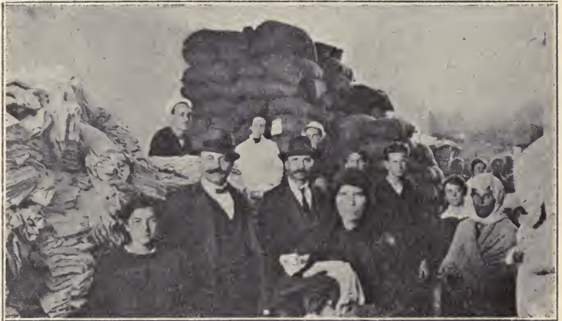
Chios; Interior of Distributing Room.
