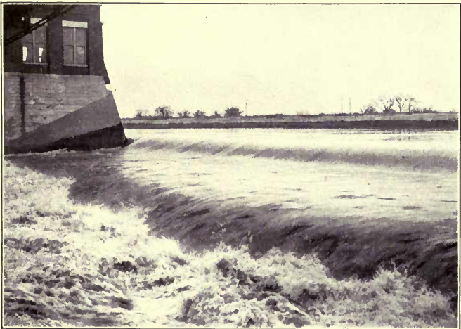
DISCHARGE OF THE CHICAGO SANITARY CANAL OVER THE BEARTRAP GATE
