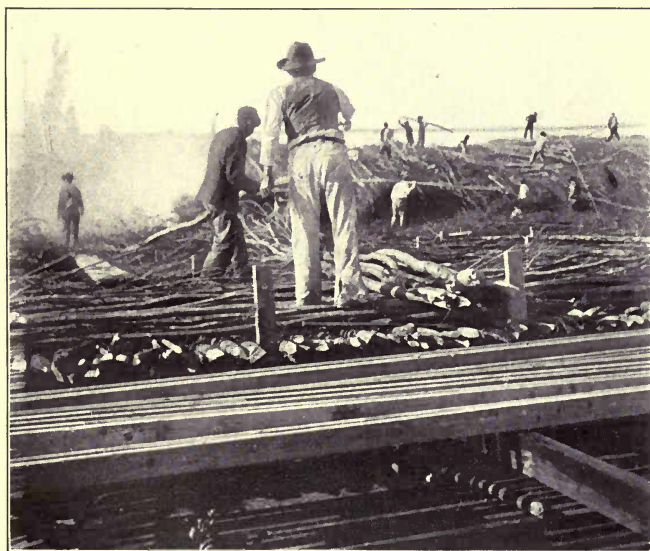
MAKING A JETTY FOUNDATION MATTRESS
