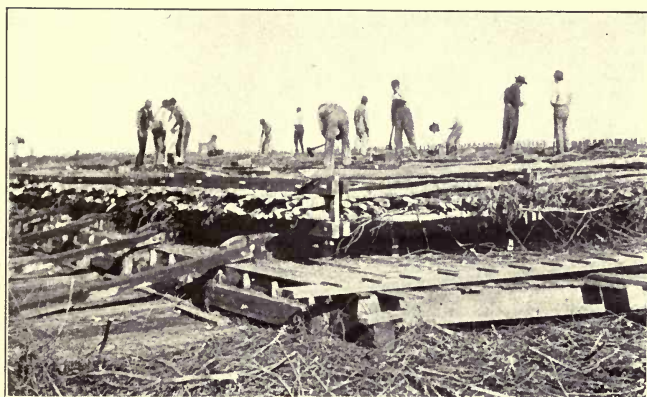
PEGGING AND FINISHING A MAT
