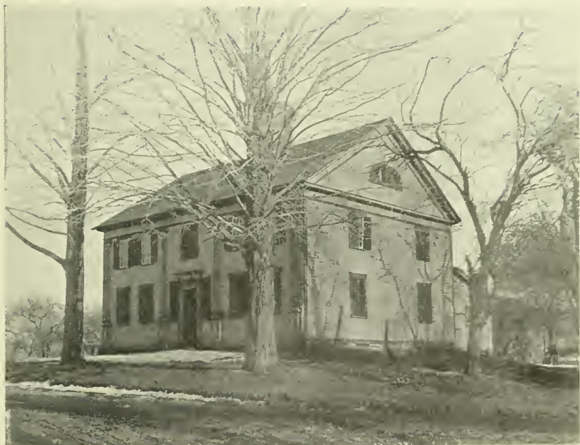
This house, built by Benj. Dyer in 1747, now known as the Page House, occupied by L. D. Dowd, is conceded by the best authorities to be the oldest house in Canton, now standing. The site of a house built a little earlier, and known as the Richard Case House, may still be seen opposite the house lately occupied by John Case, deceased.
