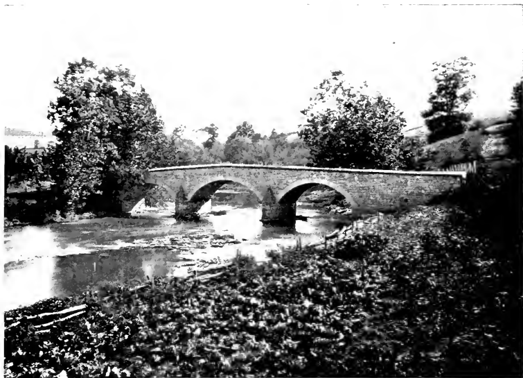
BURNSIDE BRIDGE AS IT APPEARS TO-DAY
