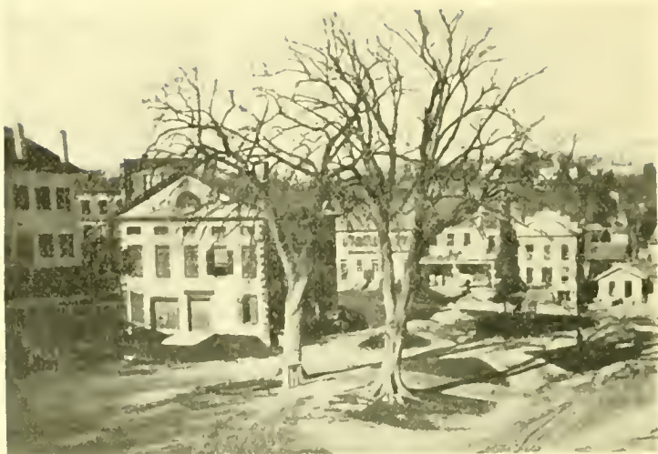
OLD TOWN HALL AND ENTRANCE TO KING STREET.
