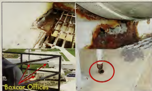
Figure 5.5-5 and 5.5-6. Examples of the seriously deteriorating infrastructure used to support the Space Shuttle Program. At left is Launch Complex 39A, and at right is the Vehicle Assembly building, both at the Kennedy Space Center.
