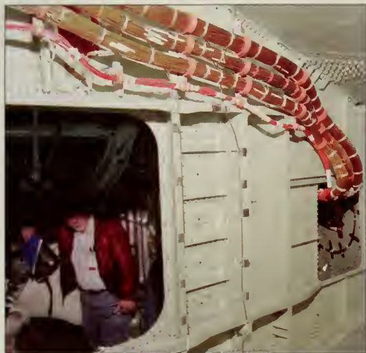
Figure 4.2-3. Typical wiring bundle inside Orbiter wing.
