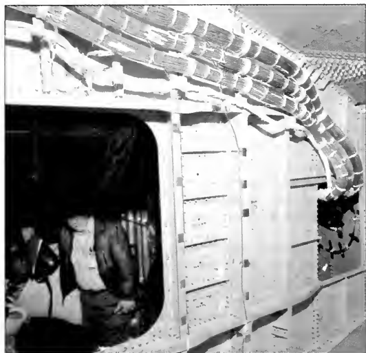
Figure 4.2-3. Typical wiring bundle inside Orbiter wing.
