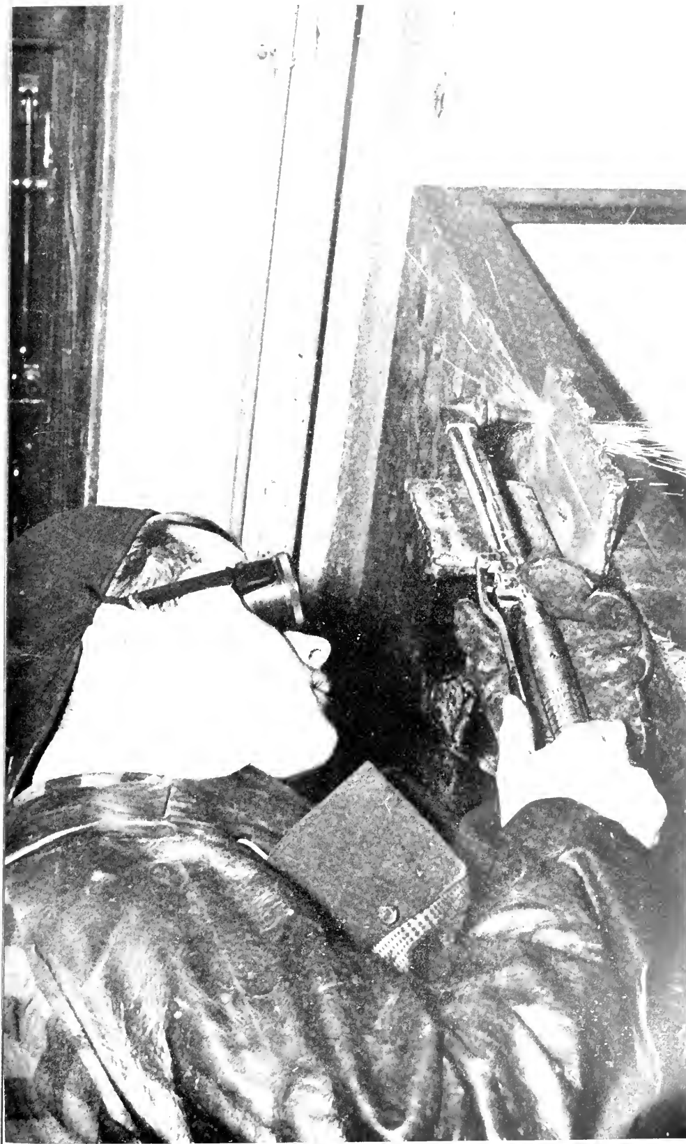
Cutting with Acetylene Torch at Welding Shop
