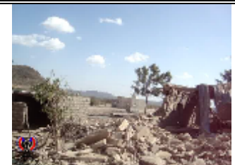
Photos of the damage left behind by the Yemini air strike, which targeted the village of Taoba in Mudia-Abyan and shelling caused the timely death of one person and wounding a number of other women in the village
