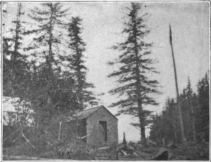
STOREHOUSE No. 1, MANZANITA COVE, WALES ISLAND, ALASKA.
