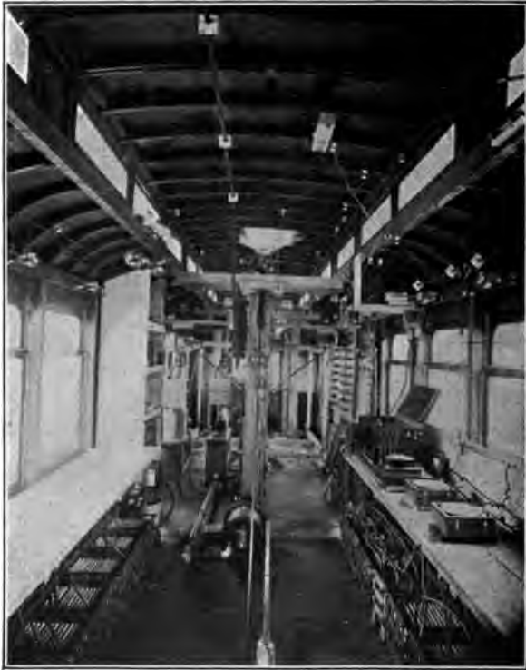
Fig. 193.—Interior View of Car "Louisiana," Looking Toward the Front from the Rear Vestibule.
