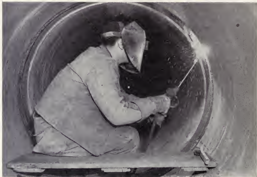
Welding steel pipe
