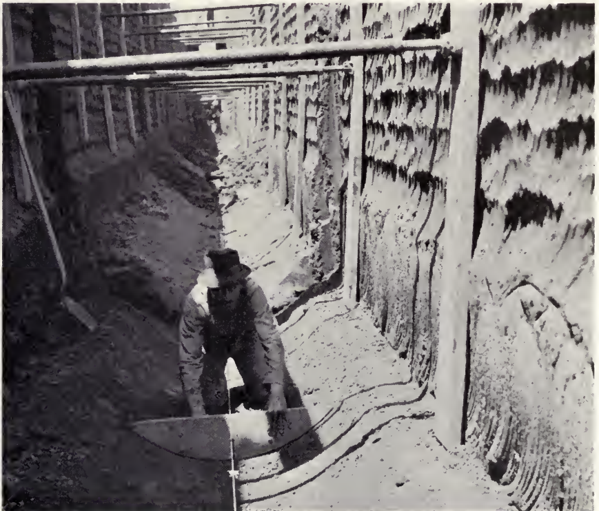
Fine grading for pipe line
