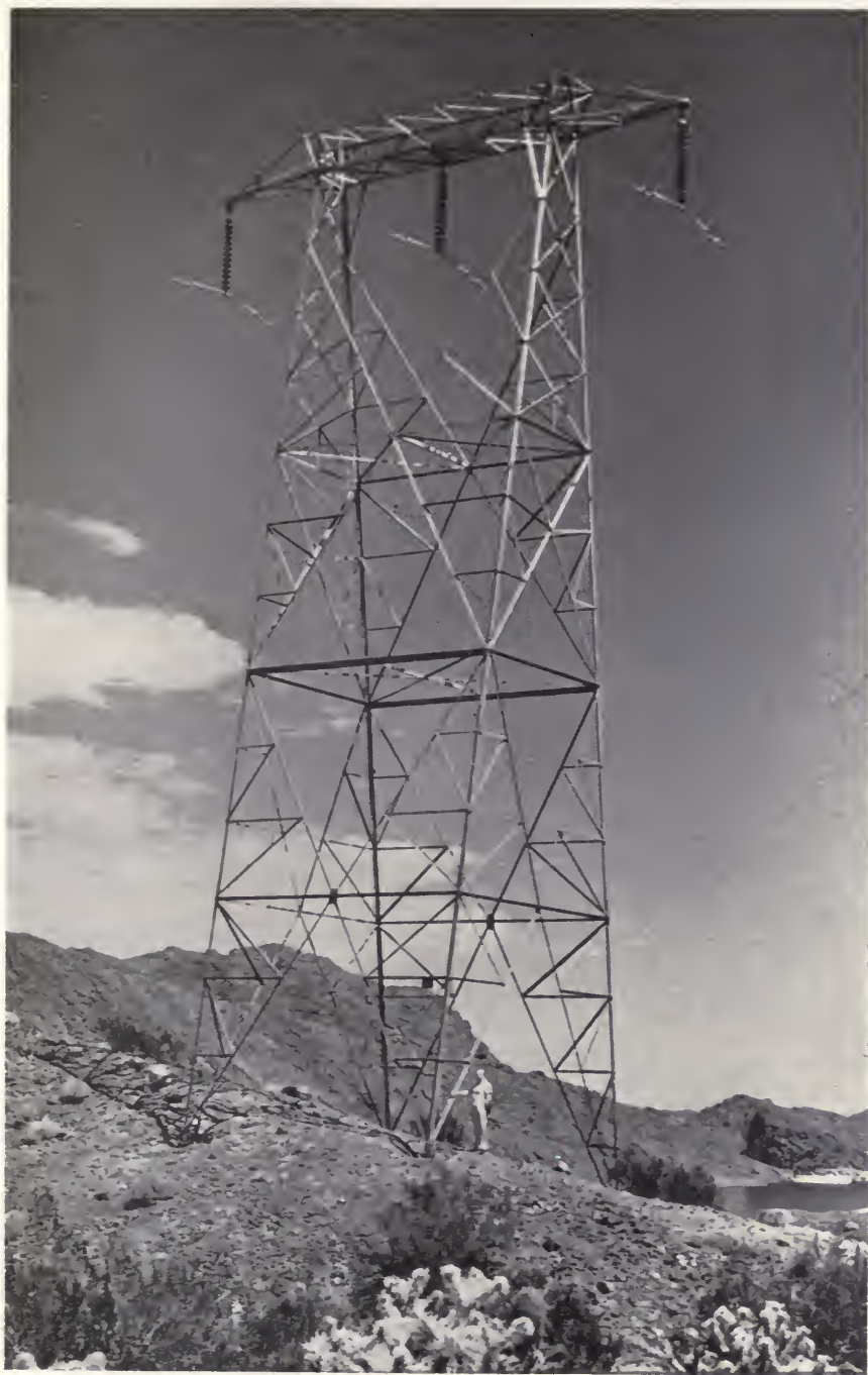
Tower on 230-kilovolt transmission line
