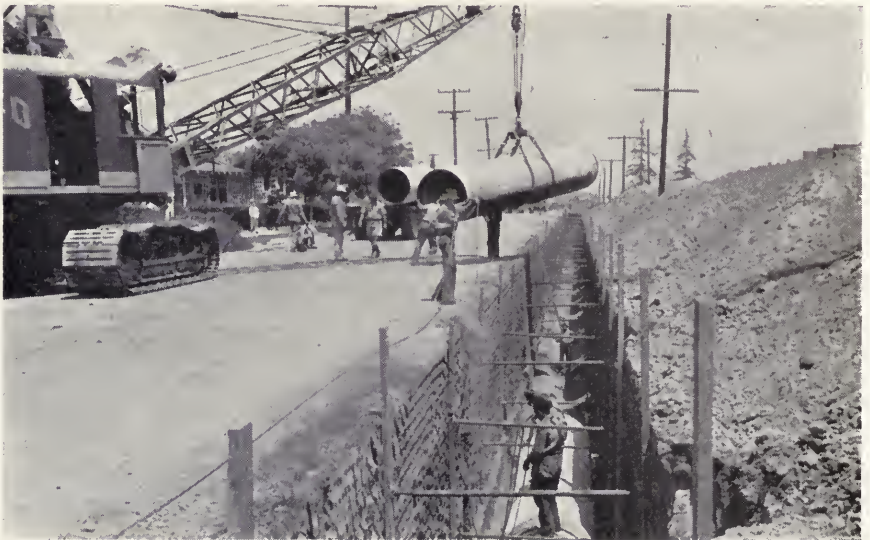
Laying steel pipe
