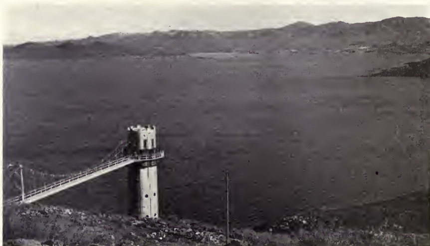
Outlet tower at Lake Mathews
