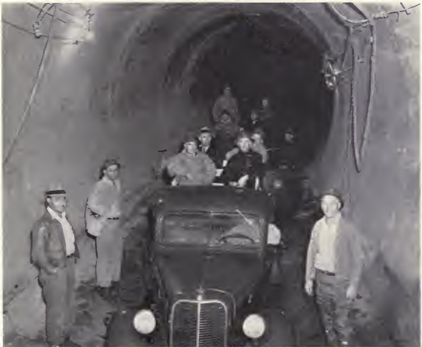
Official inspection party at San Jacinto tunnel
