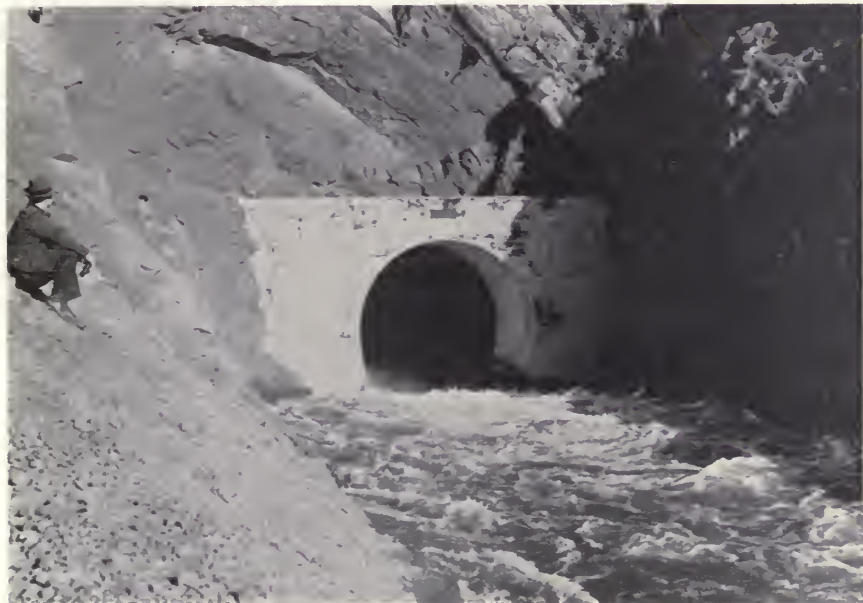
First water flowing into Copper Basin
