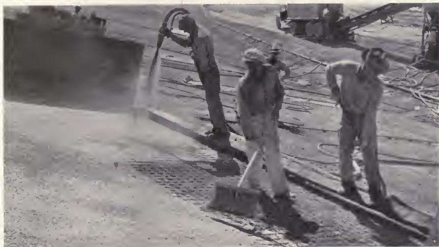
Lining reservoir with gunite
