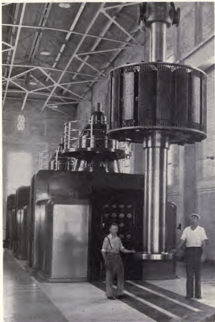
Rotor for 9000-horsepower motor at Gene
