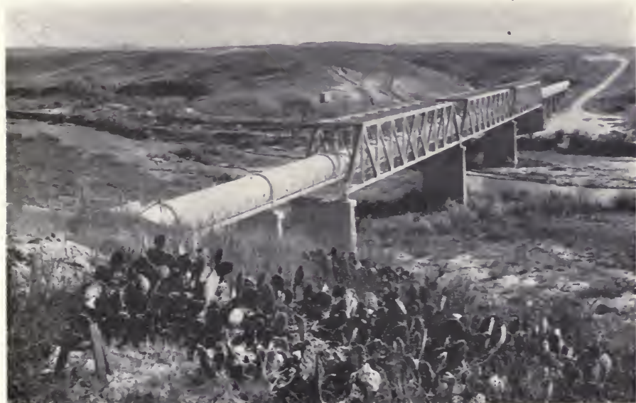
Santa Ana River crossing
