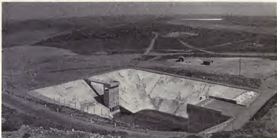
Distribution system headwork at Lake Mathews
