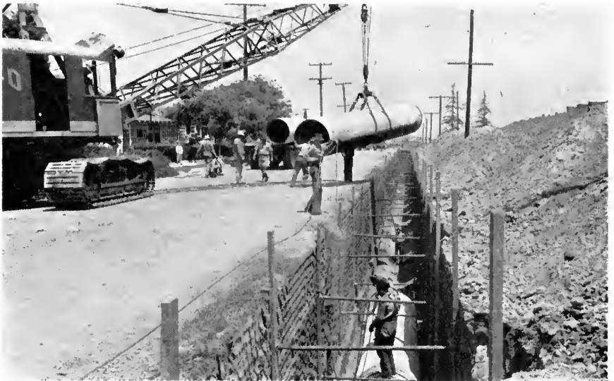
Laying steel pipe
