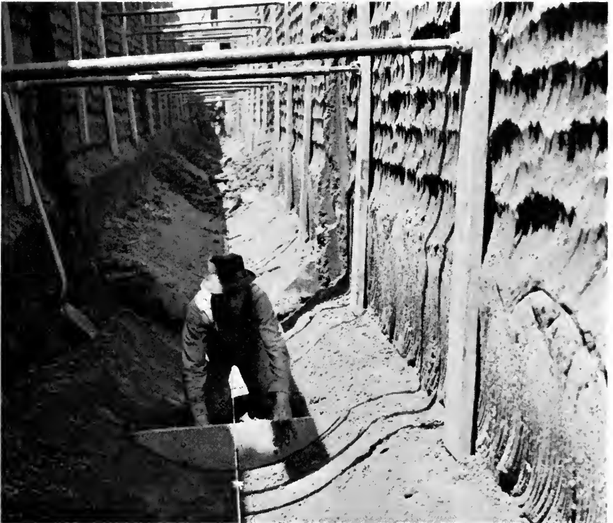
Fine grading for pipe line
