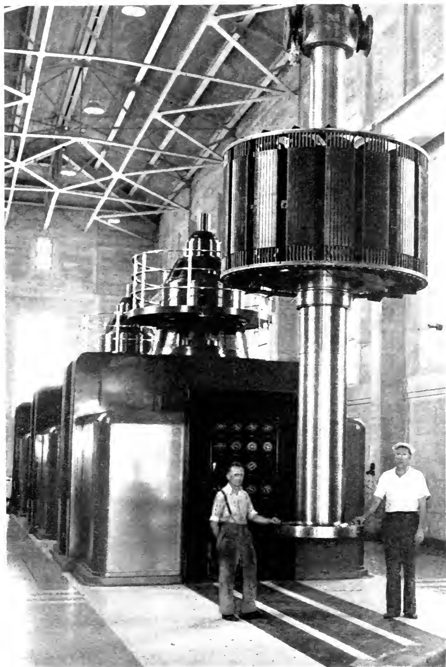
Rotor for 9000-horsepower motor at Gene
