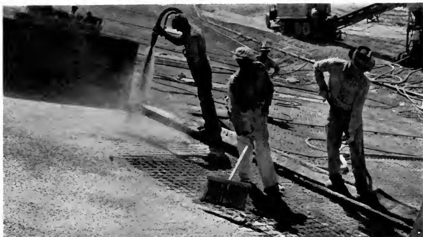
Lining reservoir with gunite
