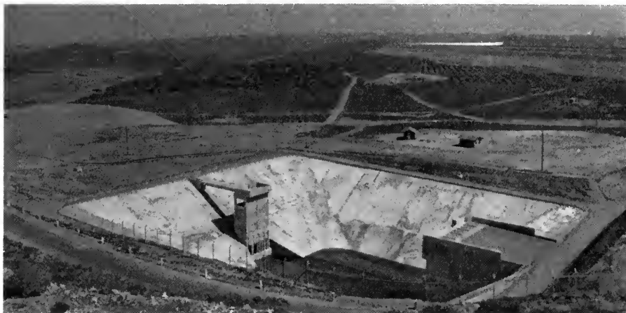
Distribution system headwork at Lake Mathews
