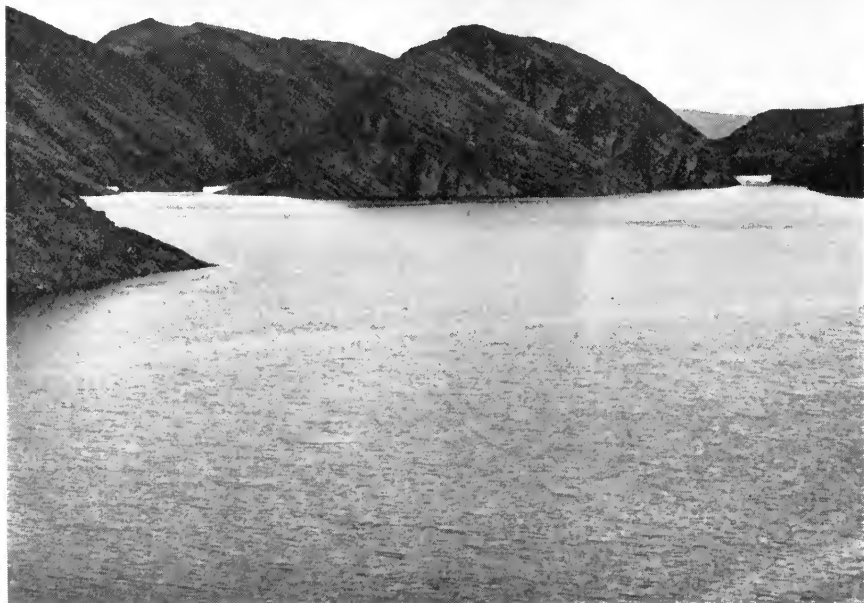
Copper Basin reservoir
