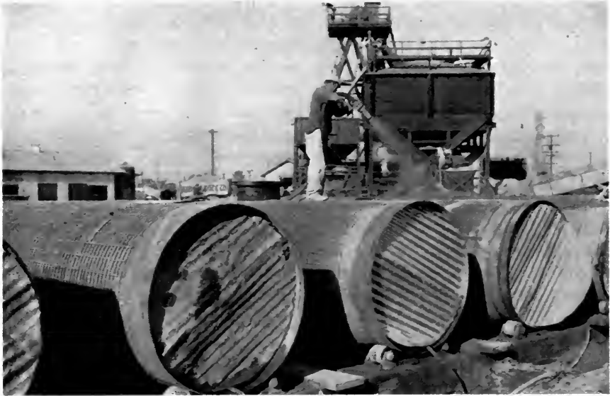
Applying guniting coating to steel pipe
