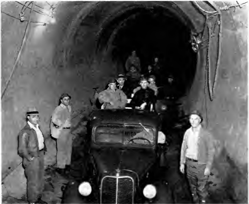
Official inspection party at San Jacinto tunnel
