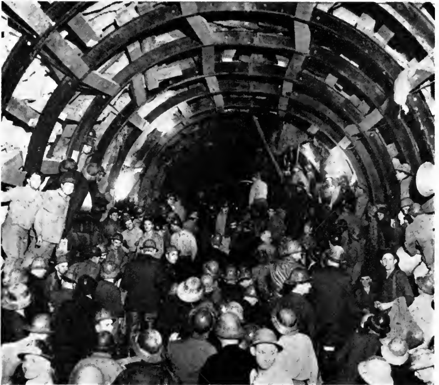
Last barrier at San Jacinto holed through
