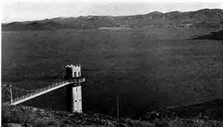
Outlet tower at Lake Mathews
