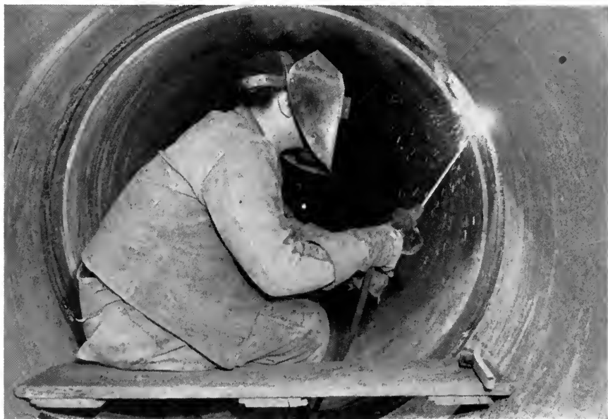
Welding steel pipe
