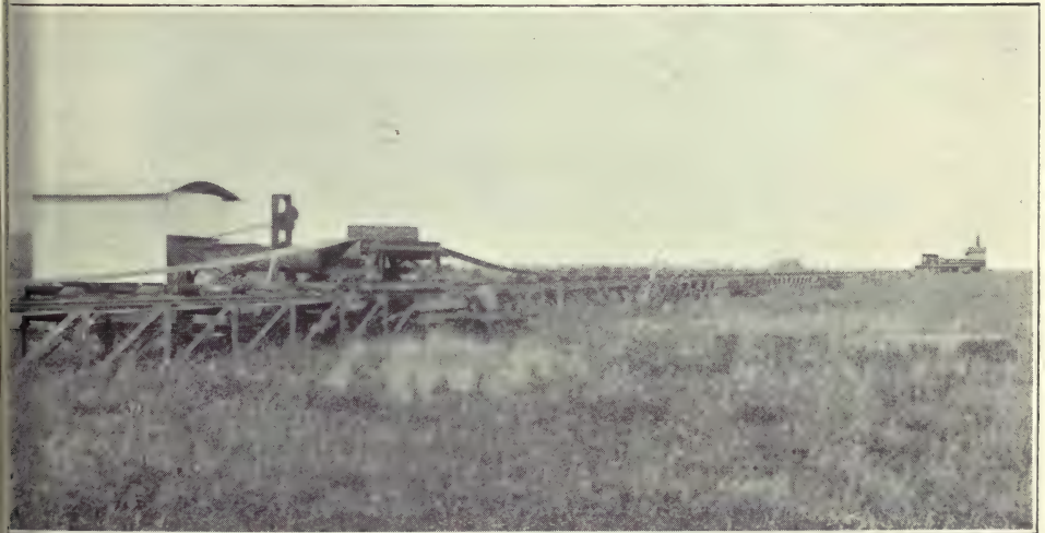
FIG. 49.—Unloading carriage on belt conveyor.
