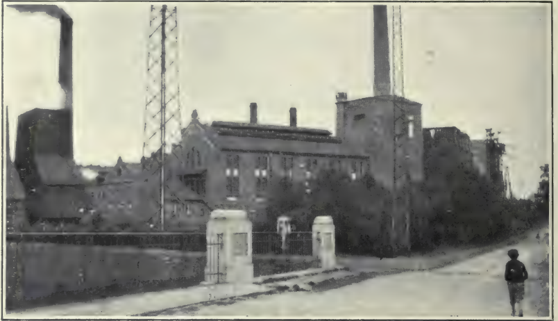
FIG. 71.—Wiesmoor Central Station, from canal bridge.
