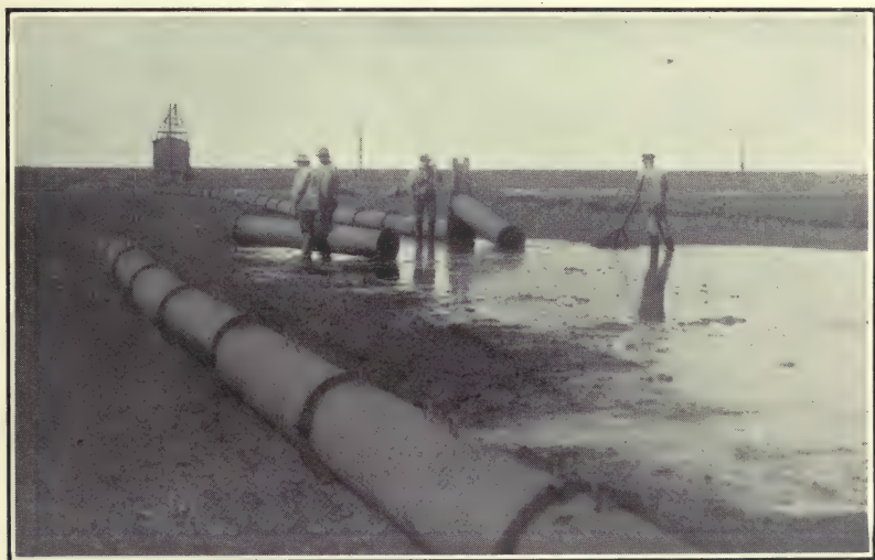
FIG. 88.—18-inch diameter pipe line.
