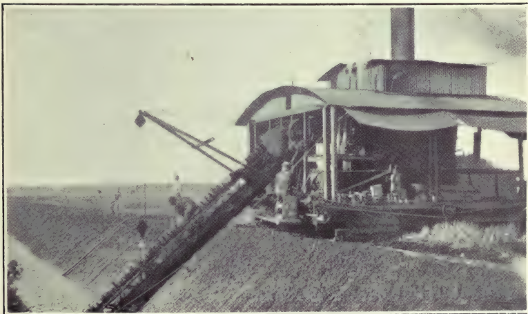
FIG. 38.—Plant No. 2, showing ladder dredge.
