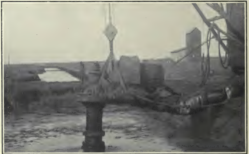
FIG. 87.—Centrifugal pump with motor over sump.
