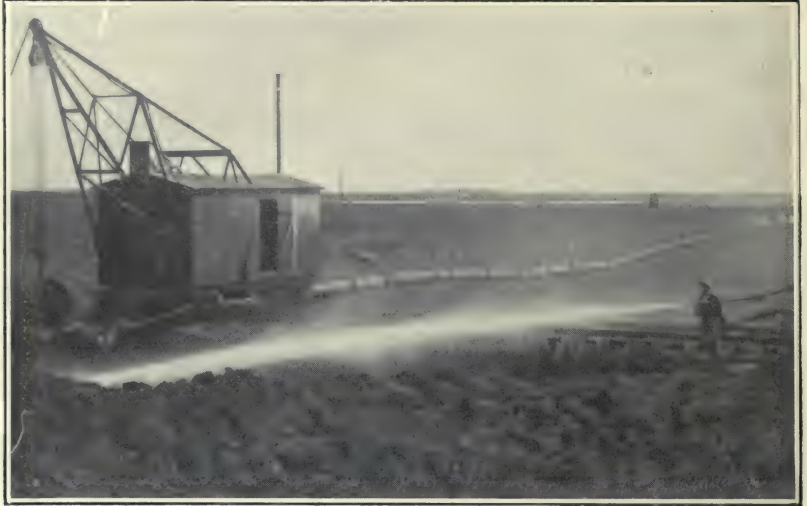
FIG. 86.—Hydro-peat process: jet, pump and pipe line.
