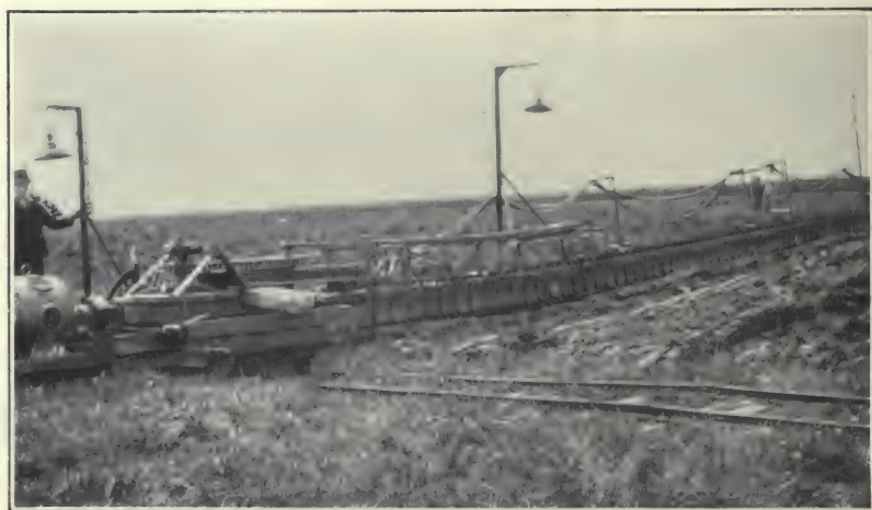
FIG. 76.—Outside end of conveyor with synchronous motor.
