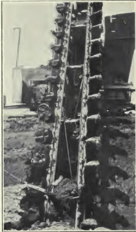
FIG. 57.—View of Wielandt dredger from trench.
