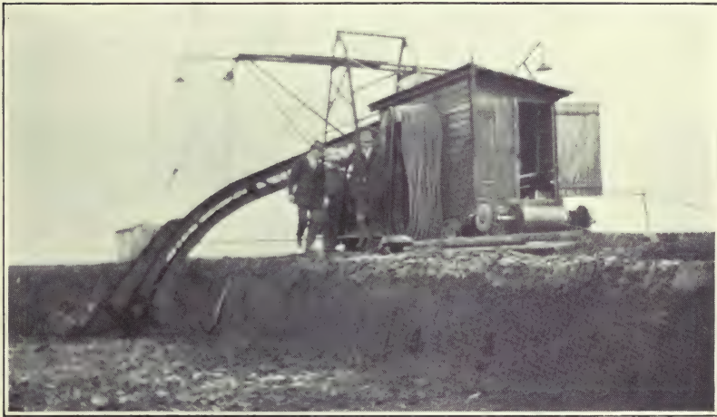
FIG. 77.—Elevator transporter machine, Wiesmoor.
