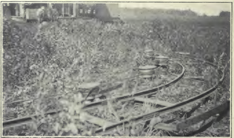
FIG. 36.—Curve at corner of spreading track.
