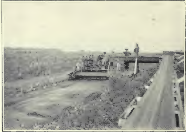
FIG. 53.—Spreader and belt shortly after erection, before cutting knives were added.
