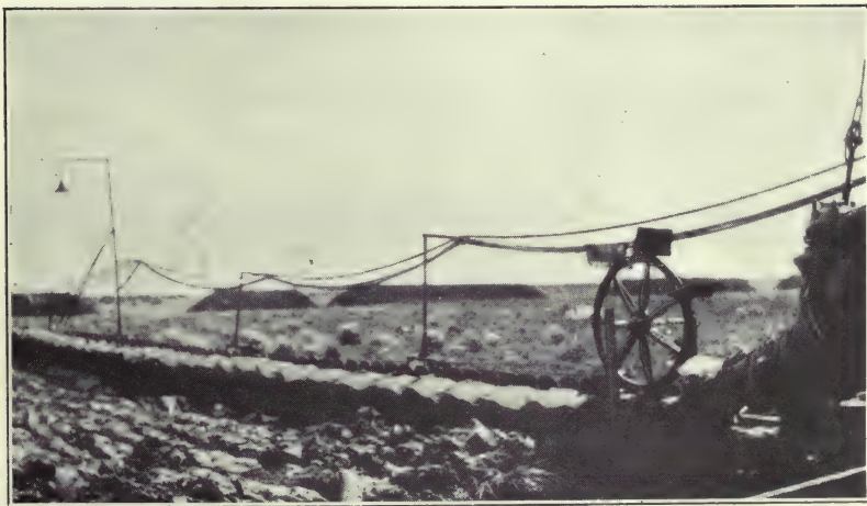
FIG. 74.—Cross-cutting device and transporter loaded with peat.
