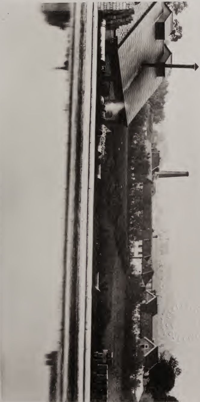
View at sewage farm, Wimbledon, England, 1885. A precipitation tank is in foreground. The fields beyond are occasionally used for filtration
