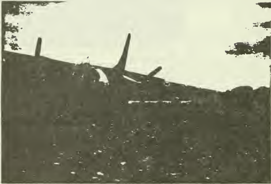
DAMAGED PROJECT DEMOCRACY C-123K # C-135 After Landing at Santa Elena Facility September 12, 1986
