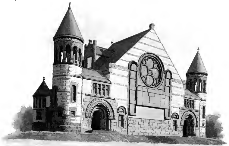
ALEXANDER COMMENCEMENT HALL.
