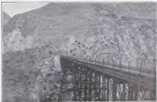
FIG. 3.—OROYA FEVER BRIDGE IN THE ANDES MOUNTAINS.
