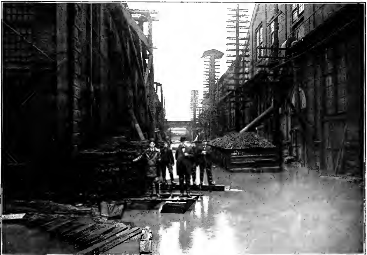
FLOOD OF MARCH 15, 1907. Plant of the Allegheny County Light Co.
