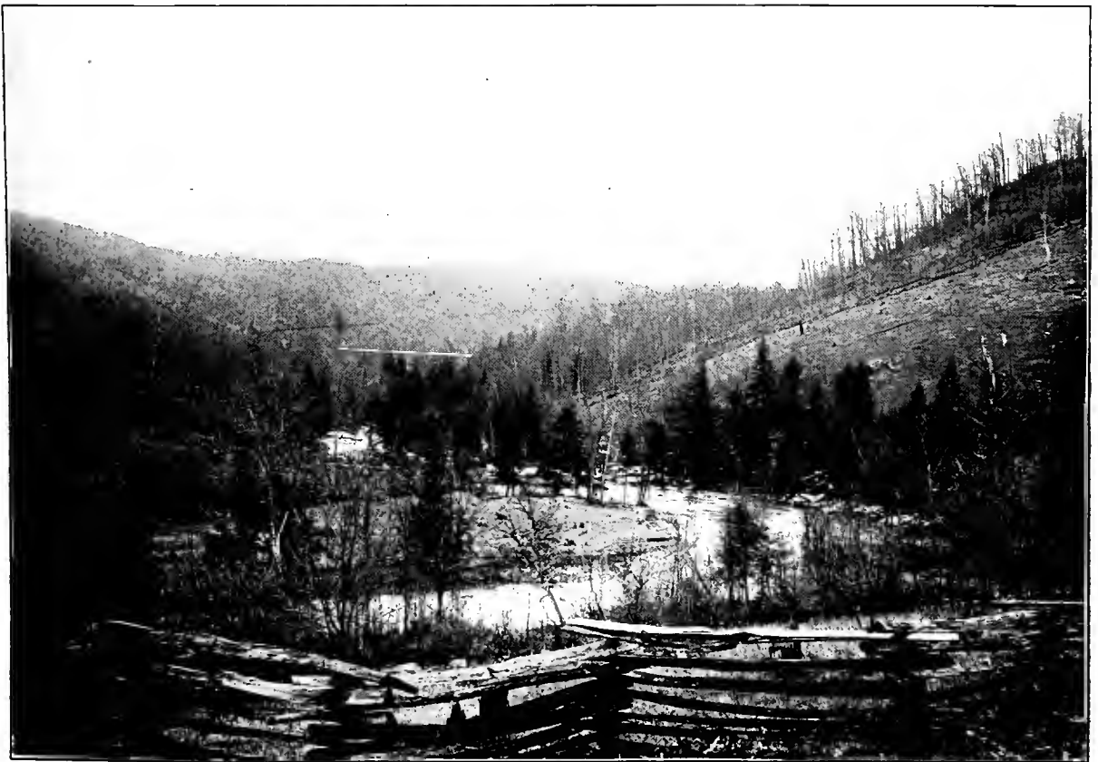
SANDY CREEK, W. VA., DECEMBER, 1910. View down stream, showing crest of proposed dam.
