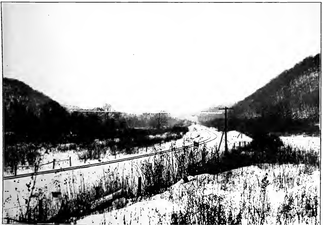
FRENCH CREEK, PA., DECEMBER, 1910. View up stream, showing crest of proposed dam.
