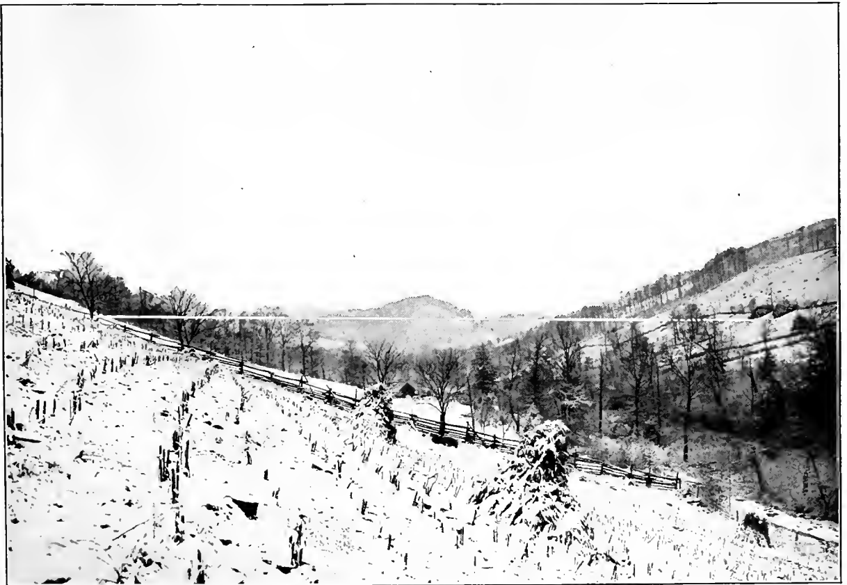
TETERS CREEK, W. VA., NOVEMBER, 1910. View down stream, showing crest of proposed dam.
