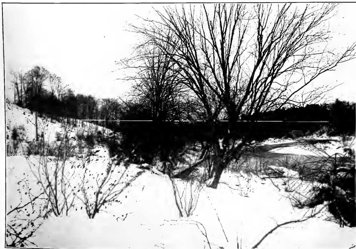
NORTH BRANCH FRENCH CREEK, PA., DECEMBER, 1910. View down stream, showing crest of proposed dam.
