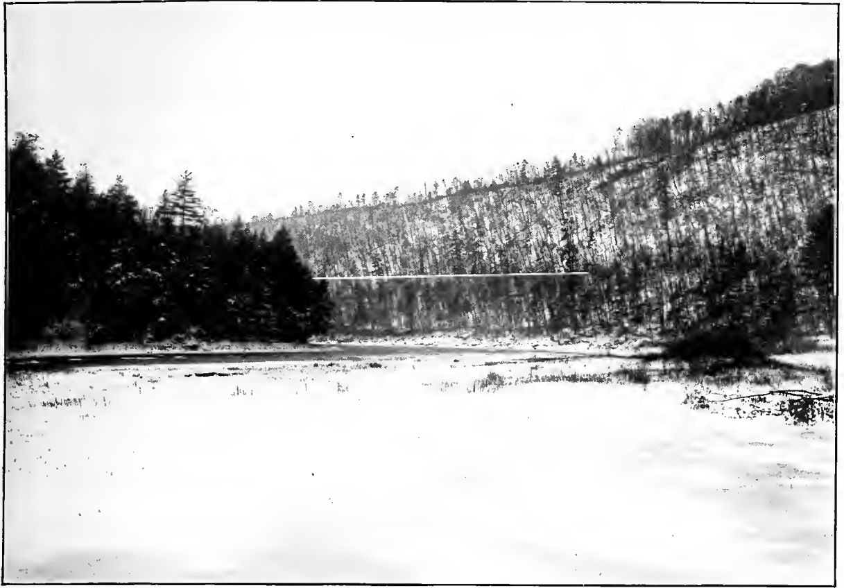
CLARION RIVER, PA., OCTOBER, 1910. View up stream, showing crest of proposed Dam No. 2.
