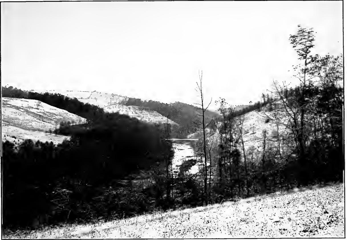
BUCKHANNON RIVER, W. VA., NOVEMBER, 1910. View up stream, showing crest of proposed dam.
