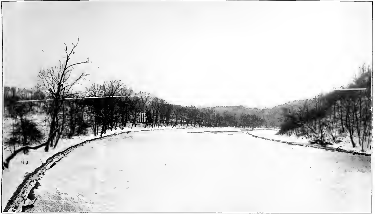
CROOKED CREEK, PA., FEBRUARY, 1911. View up stream, showing crest of proposed dam.
