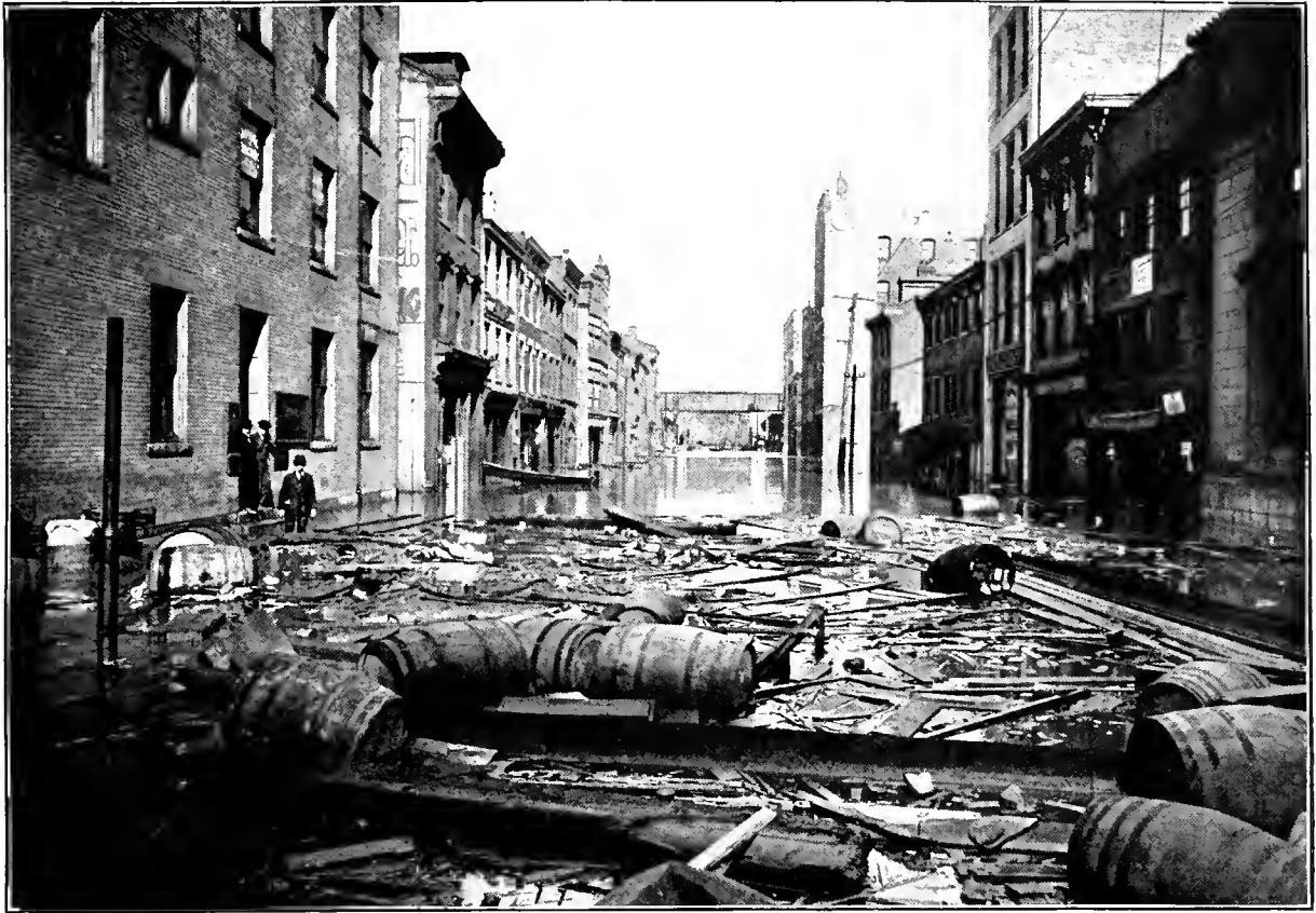
FLOOD OF MARCH 15, 1907. Ninth Street, looking north from Penn Avenue. Deposit left by high water.
