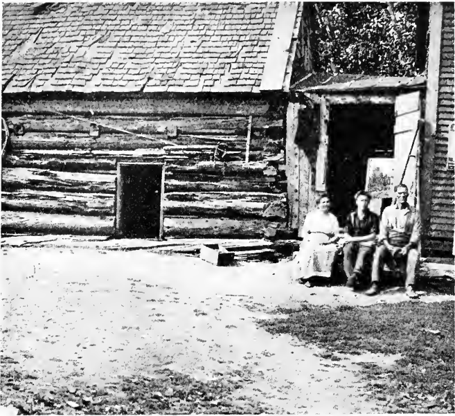
Note the low doorway used by three generations before the modern frame structure was added.
