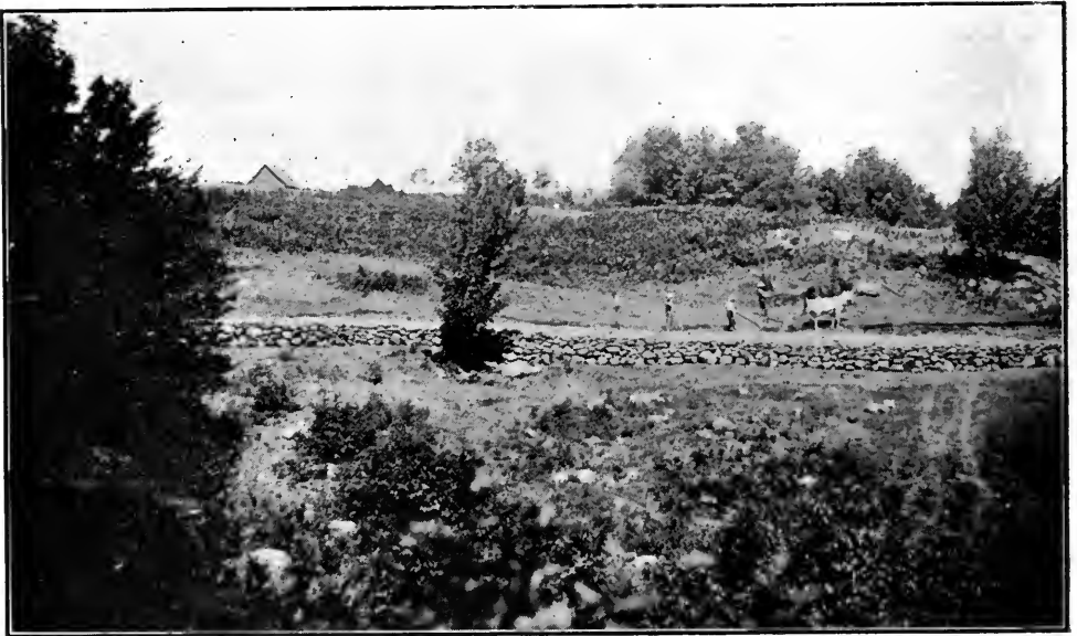
Road construction—Muskoka District.
