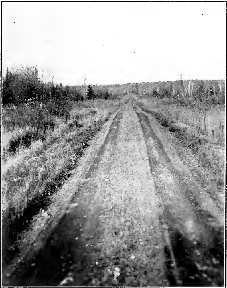
A view of the International or Scott Highway between Fort William and Pigeon River, showing road surfaced with shale and gravel.
