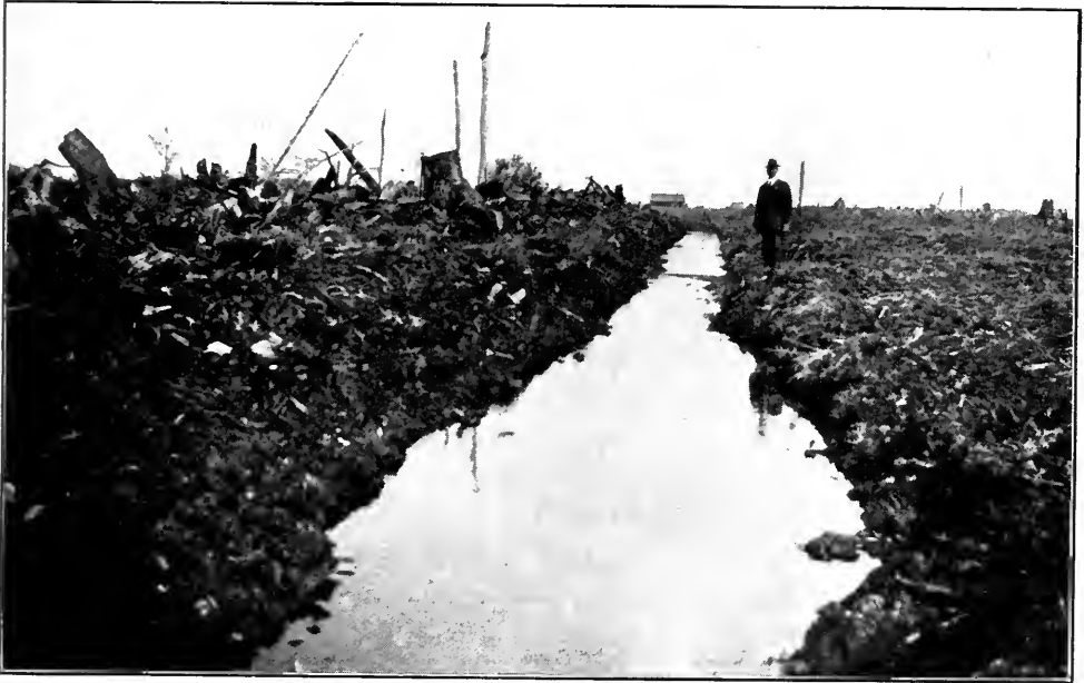
Drain in swamp constructed entirely by means of blasting powder.
