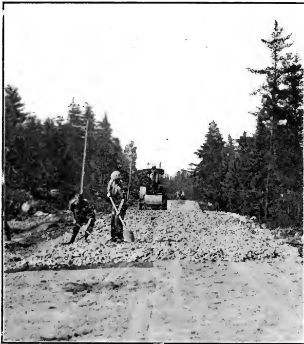
Macadam road under construction.
