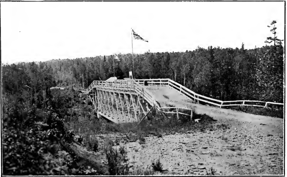
International Bridge—Pigeon River, Port Arthur-Duluth Road.
