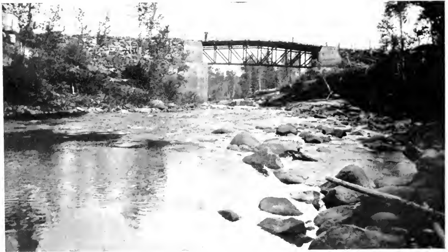
McKenzie River Bridge, Northern Ontario.
