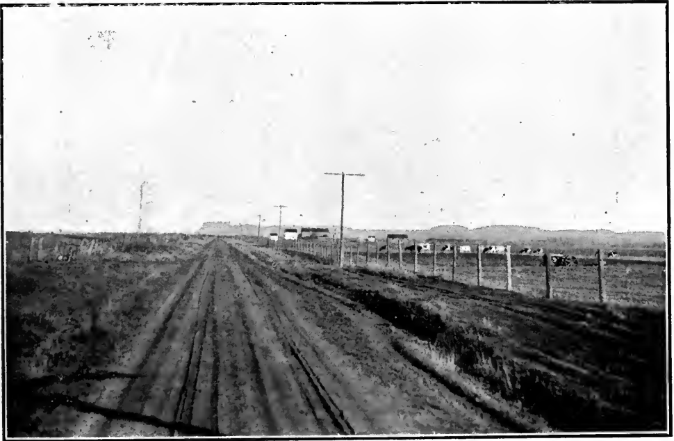
A view along the Trunk Road through the Slate River Valley, south-west of Fort William.
