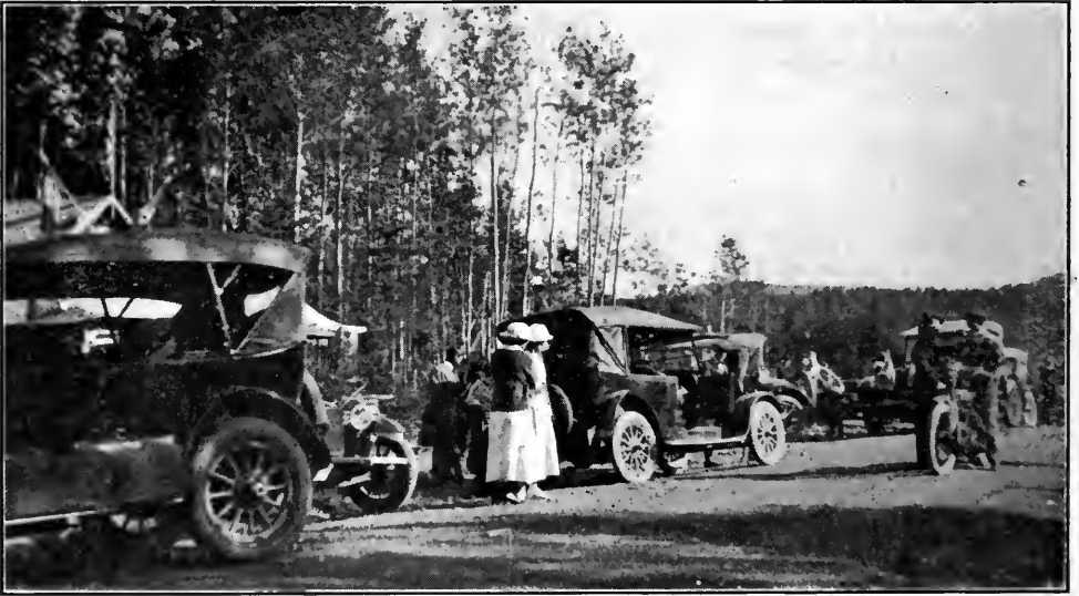
Sunday traffic—International Bridge, Pigeon River—Port Arthur and Duluth Railway.
