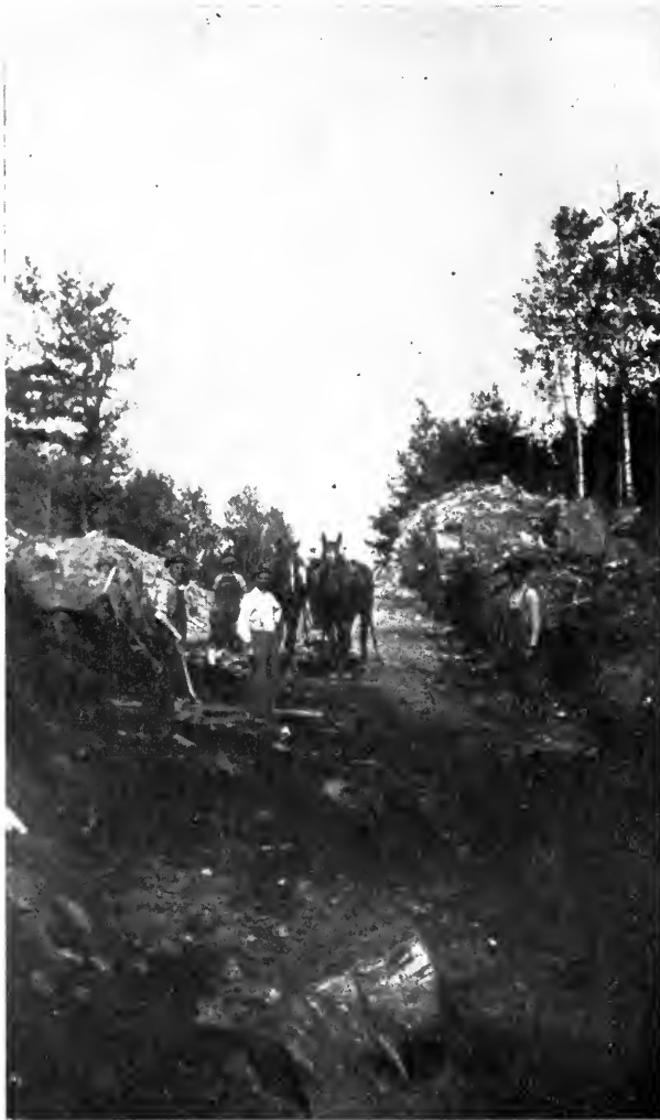
Road Construction in Muskoka.
