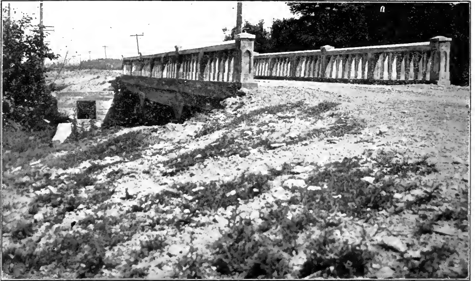
Bar River Bridge—Algoma District.
