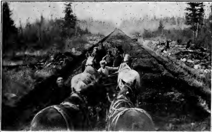
Opening a new road, Rainy River District
