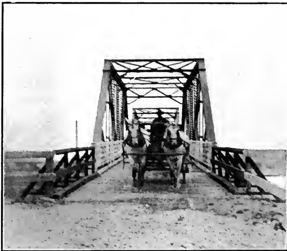
Steel Bridge—Timmins, Mattagami River.
