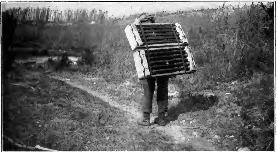
☒ Packing Survey Posts.
