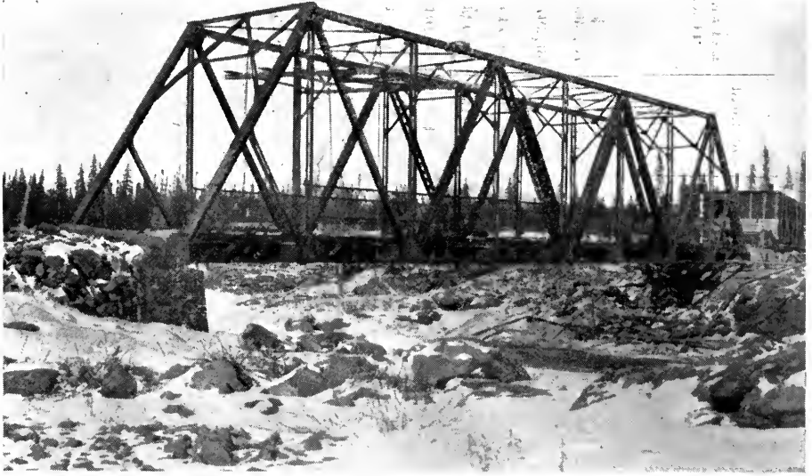
Steel bridge at Kapuskasing; erected 1919.
