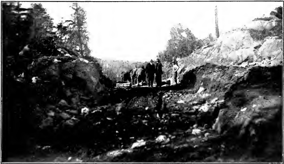
Pioneer road through rock cut, Muskoka District.
