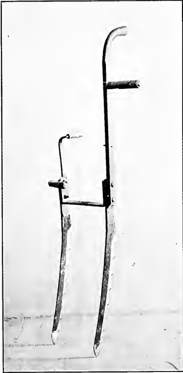
a. Modified hay knife for recutting ditches in salt marsh.
