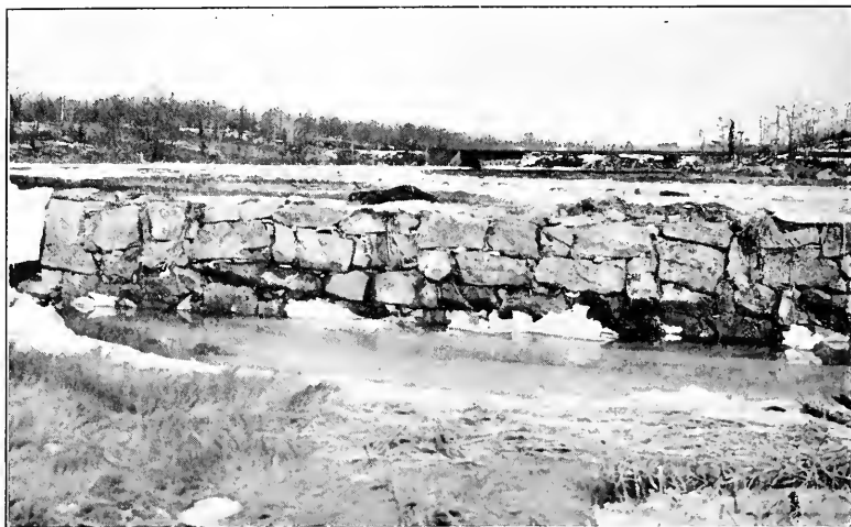
b. New dike, Stony Creek.
