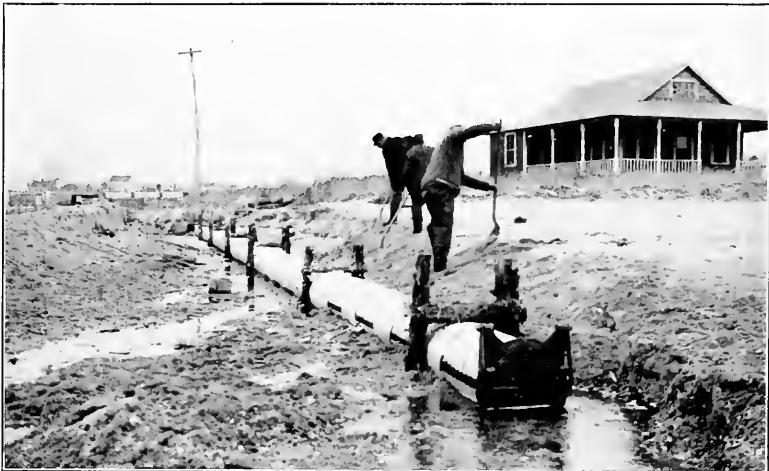
c. Installing a metal culvert through a sand beach to drain the marsh beyond, Westbrook.
