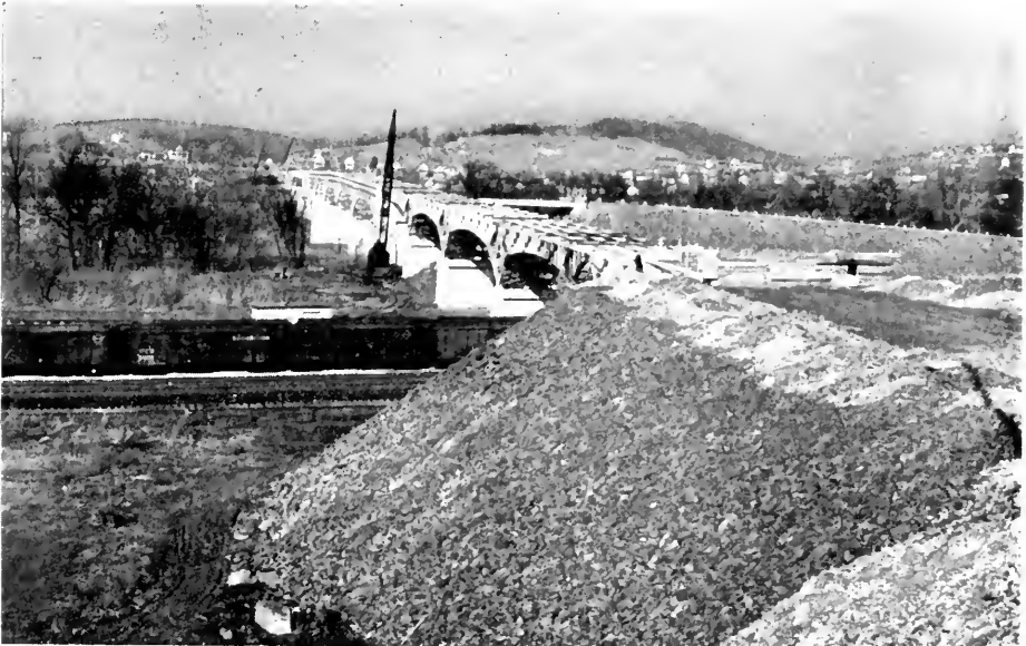
BRIDGE OVER POTOMAC RIVER AT HANCOCK LOOKING FROM WEST VIRGINIA TOWARD MARYLAND
