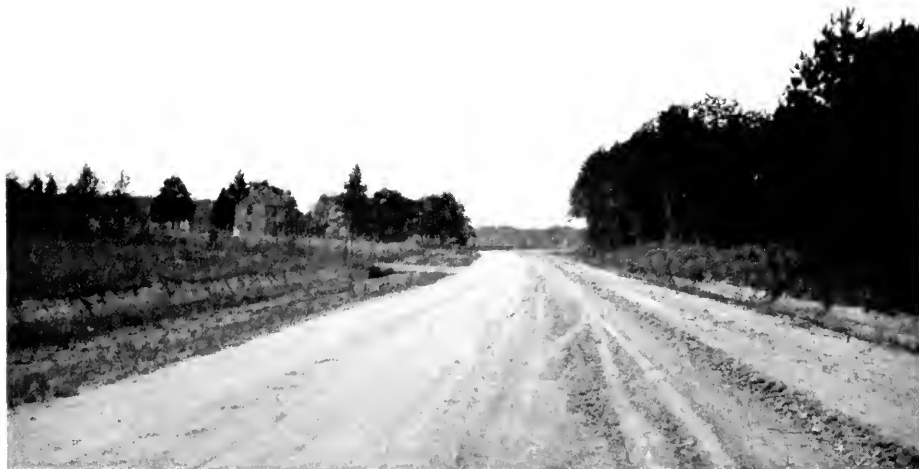
VENTON CHURCH TO MOXIE—SOMERSET COUNTY BEFORE AND AFTER IMPROVEMENT
