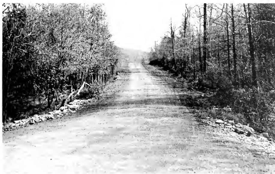
HOYES RUN ROAD GARRETT COUNTY BEFORE AND AFTER IMPROVEMENT
