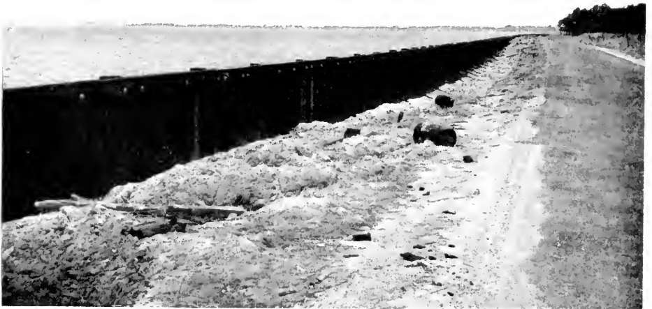
BULKHEAD ALONG STATE HIGHWAY—ST. GEORGE'S ISLAND ST. MARY'S COUNTY
