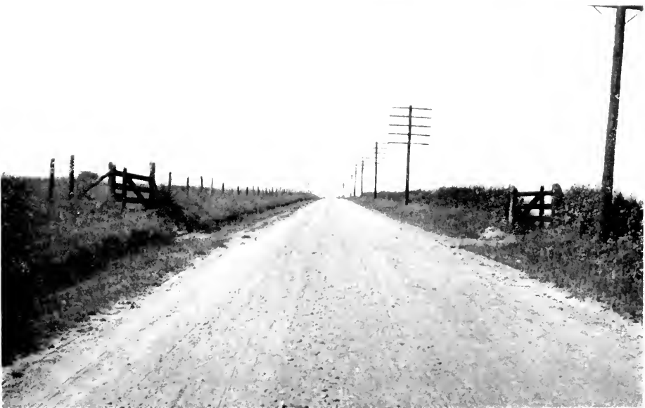
BOHEMIA CREEK ROAD—CECIL COUNTY BEFORE AND AFTER IMPROVEMENT
