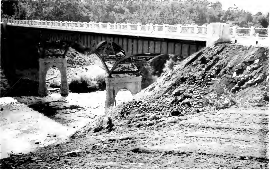
BRIDGE OVER LICKING CREEK—NATIONAL HIGHWAY WASHINGTON COUNTY
