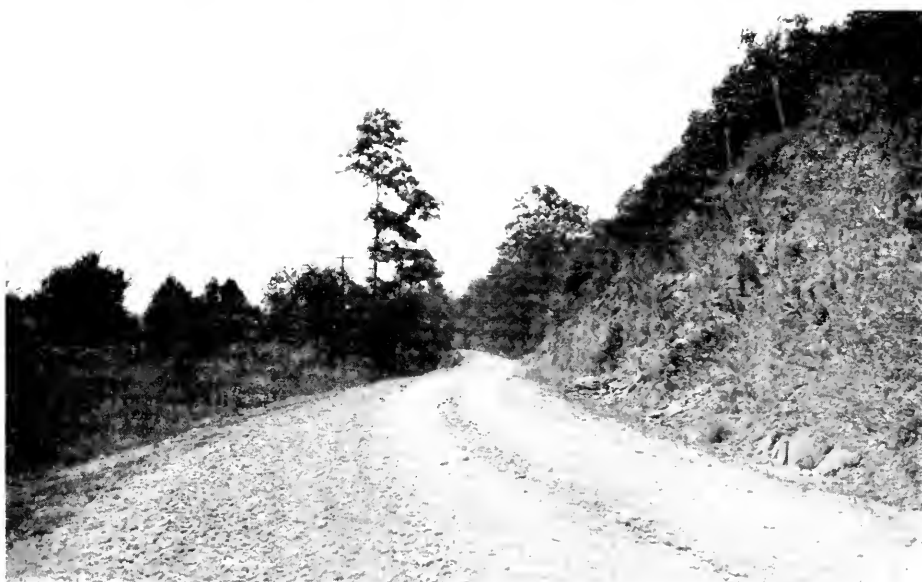
COMUS-HYATTSTOWN ROAD - MONTGOMERY COUNTY BEFORE AND AFTER IMPROVEMENT
