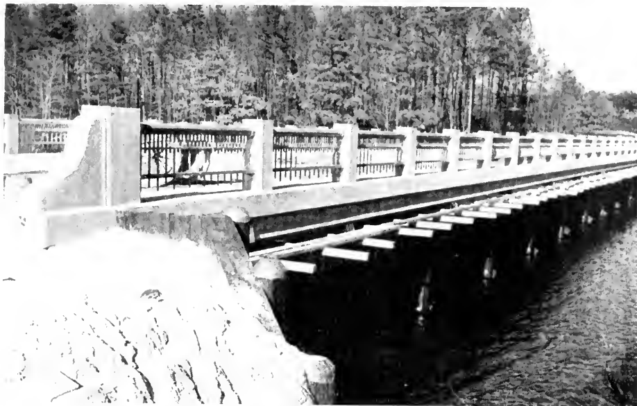
BRIDGE OVER TONYTANK POND—WICOMICO COUNTY
