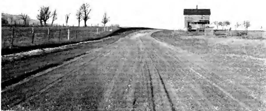
OLD FREDERICK ROAD—FREDERICK COUNTY BEFORE AND AFTER IMPROVEMENT
