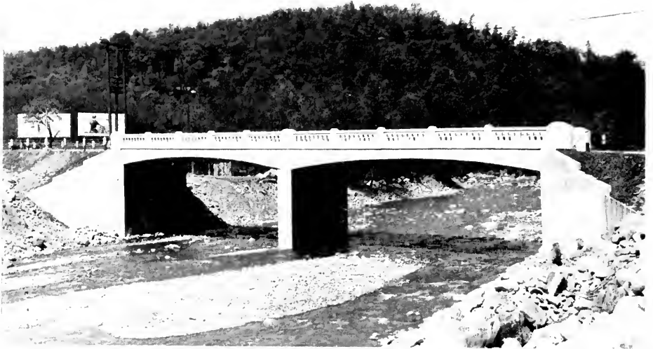
BRIDGE OVER SAVAGE RIVER AT BLOOMINGTON—GARRETT COUNTY
