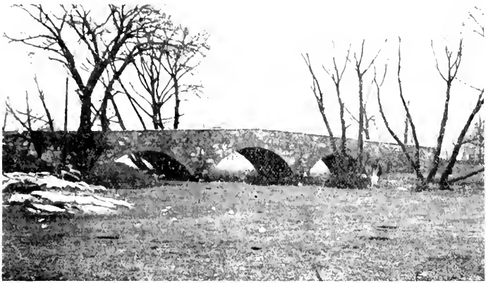
OLD STONE MASONRY ARCH BRIDGE OVER ANTIETAM CREEK ON ROAD FROM HAGERSTOWN TO LEITERSBURG. WASHINGTON COUNTY
