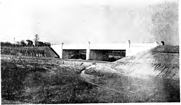
THE COMPLETED GRADE SEPARATION STRUCTURE NEAR GOLDEN RING, SHOWING THE STARTING OF EROSION OF THE SLOPES
