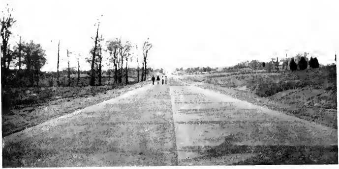
A COMPLETED SECTION OF THE LYONS CORNER-MORGANTOWN BRIDGE JOB IN CHARLES COUNTY
