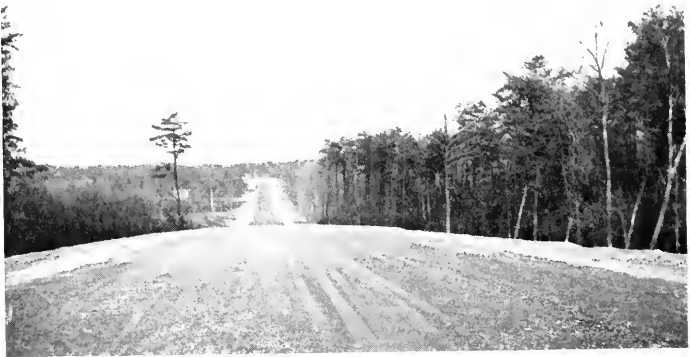
THE BOWIE RACE TRACK ROAD AFTER IMPROVEMENT
