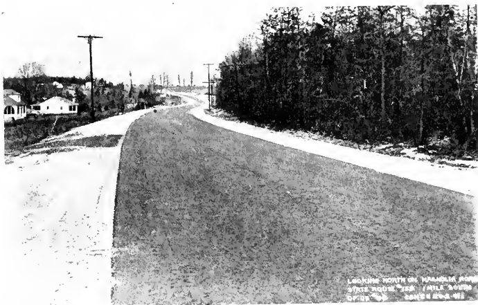
THE MAGNOLIA ROAD, ORIGINALLY CONSTRUCTED AS A SECONDARY ROAD BUT RECONDITIONED TO SERVE AS AN ACCESS HIGHWAY
