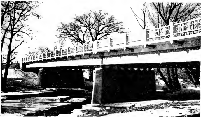
NEW BRIDGE OVER ANTIETAM CREEK ON HAGERSTOWN-LEITERSBURG ROAD, REPLACING OLD STONE ARCH. WASHINGTON COUNTY
