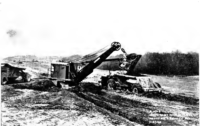
GRADING EQUIPMENT AT WORK ON THE NORTH POINT ROAD
