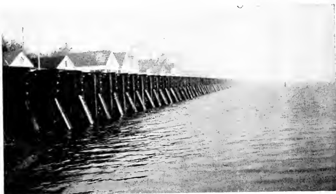
THE BULKHEAD AT NORTH BEACH IN CALVERT COUNTY
