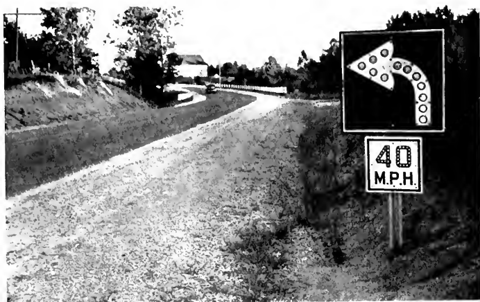
THE "SAFE SPEED" SIGN USED TO ELIMINATE THE "SURPRISE ELEMENT" ON SHARP CURVES
