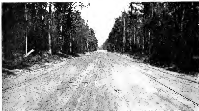
AN UNPAVED SECTION OF GRADED AND WIDENED COUNTY HIGHWAY IN WICOMICO COUNTY
