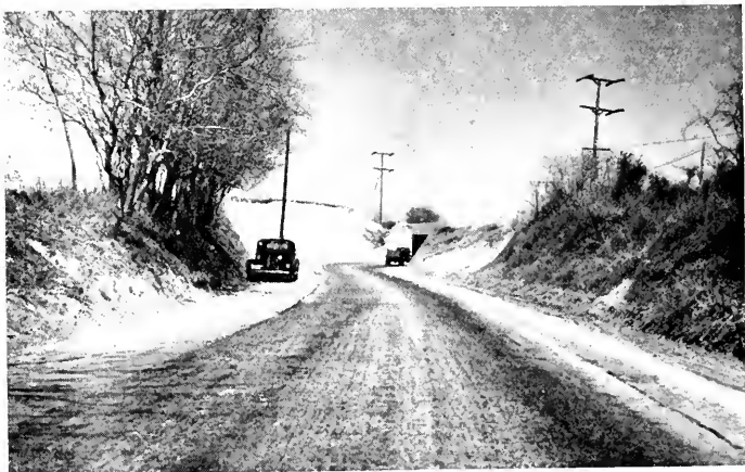
A VERY DANGEROUS "BOTTLENECK" SOUTH OF PUMPHREY ON THE ROAD TO FORT MEADE CAUSED BY A REVERSE AND AN UNDERPASS OF THE OLD W. B. & A. R. R.
