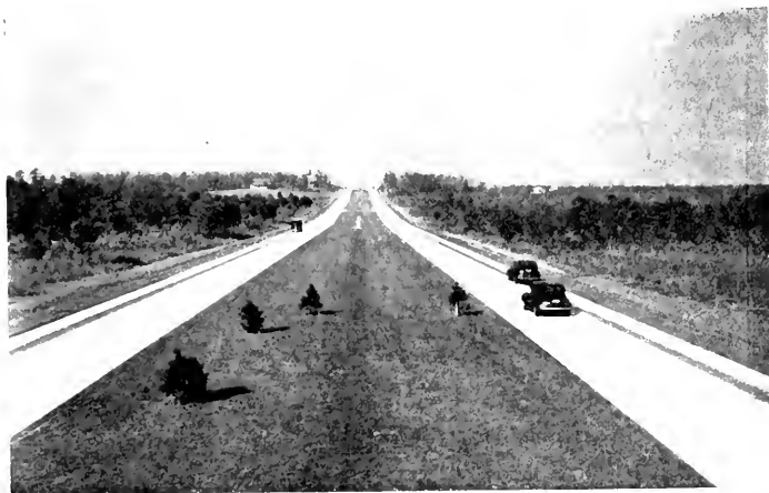
A SECTION OF THE GOVERNOR RITCHIE HIGHWAY SOUTH OF GLEN BURNIE
