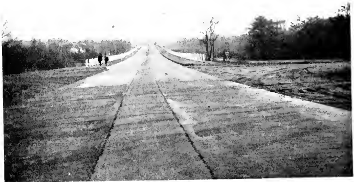
THE EAST APPROACH TO THE LANDOVER GRADE ELIMINATION PROJECT IN PRINCE GEORGE'S COUNTY
