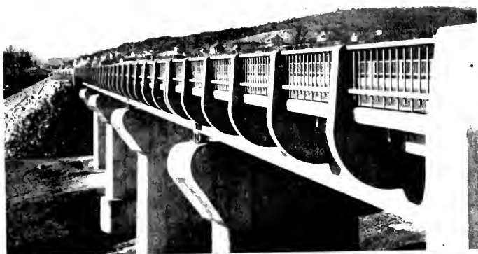
NEW BRIDGE OVER TONOLOWAY CREEK ON A RELOCATION OF U. S. ROUTE 40 JUST EAST OF HANCOCK, WASHINGTON COUNTY
