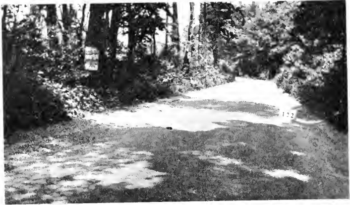
THE BOWIE RACE TRACK ROAD BEFORE IMPROVEMENT
