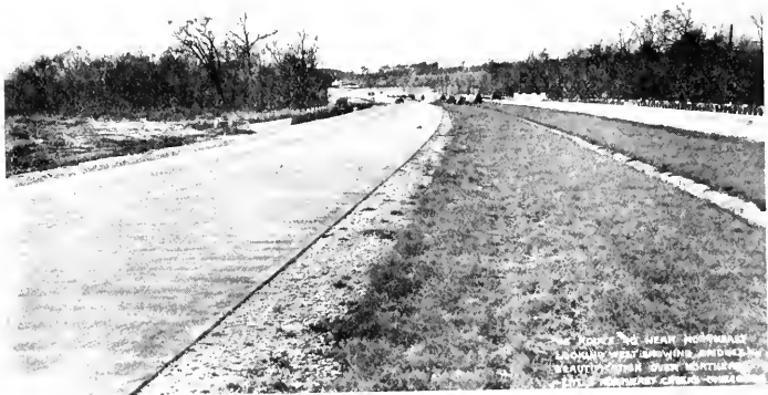
THE RELOCATED ROUTE 40 EAST OF NORTHEAST, SHOWING PROVISIONS FOR CENTER DRAINAGE, THE GRAVEL STABILIZING OF THE SHOULDERS ON EACH SIDE OF THE PAVING, THE TURN-OUT AREAS NEAR THE BRIDGE, AND THE RECENTLY COMPLETED ROADSIDE DEVELOPMENT IN THE PARK AREA
