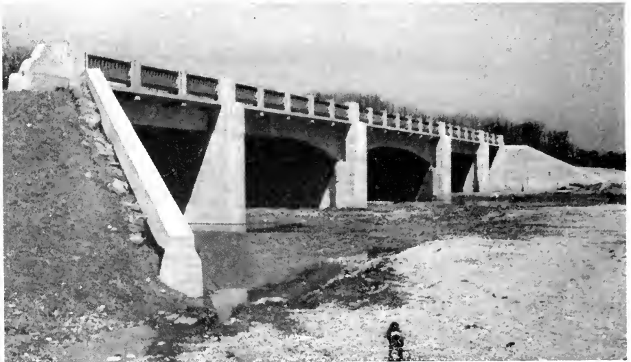
CONTINUOUS CONCRETE GIRDER BRIDGE OVER PATUXENT RIVER ON MILITARY ACCESS ROAD FROM FORT MEADE TO U. S. ROUTE 1, AT THE ANNE ARUNDEL-PRINCE GEORGE'S COUNTY LINE
