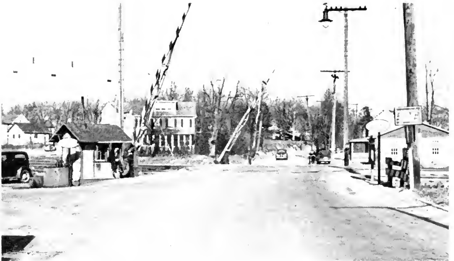
SULPHUR SPRING ROAD GRADE CROSSING OF PENNSYLVANIA RAILROAD AT ARBUTUS The elimination of these grade crossings is of major importance and the improvements are contemplated in the post-war period
