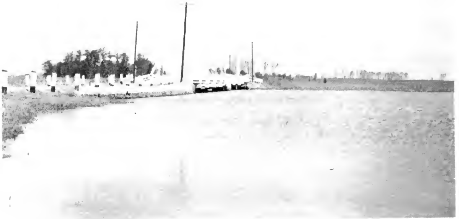
EASTERN NECK ISLAND BRIDGE BETWEEN KENT COUNTY MAINLAND AND EASTERN NECK ISLAND—BEFORE REBUILDING
