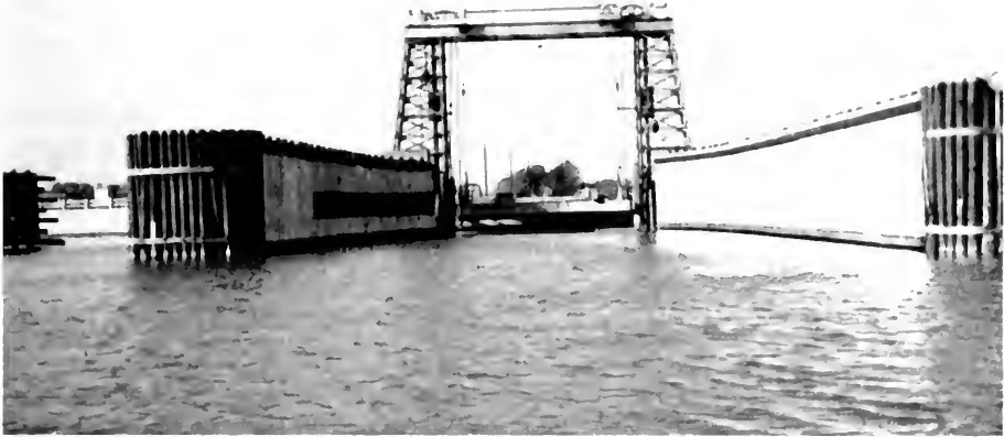
SLIP AND TRANSFER BRIDGE, SANDY POINT FERRY TERMINAL, ANNE ARUNDEL COUNTY
