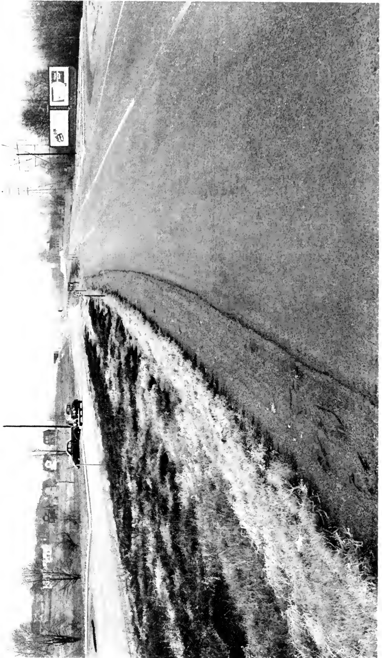
AN INTERSECTION AT GRADE BY CHANNELLING ON THE BITUMINOUS CONCRETE SURFACING BETWEEN EASTERN AVENUE AND SPARROWS POINT ON THE NORTH POINT ROAD
