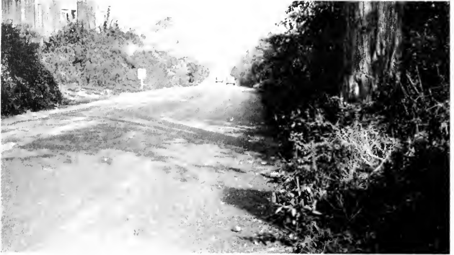
A POINT ON THE DAVIDSONVILLE ROAD BEFORE WIDENING AND RESURFACING
