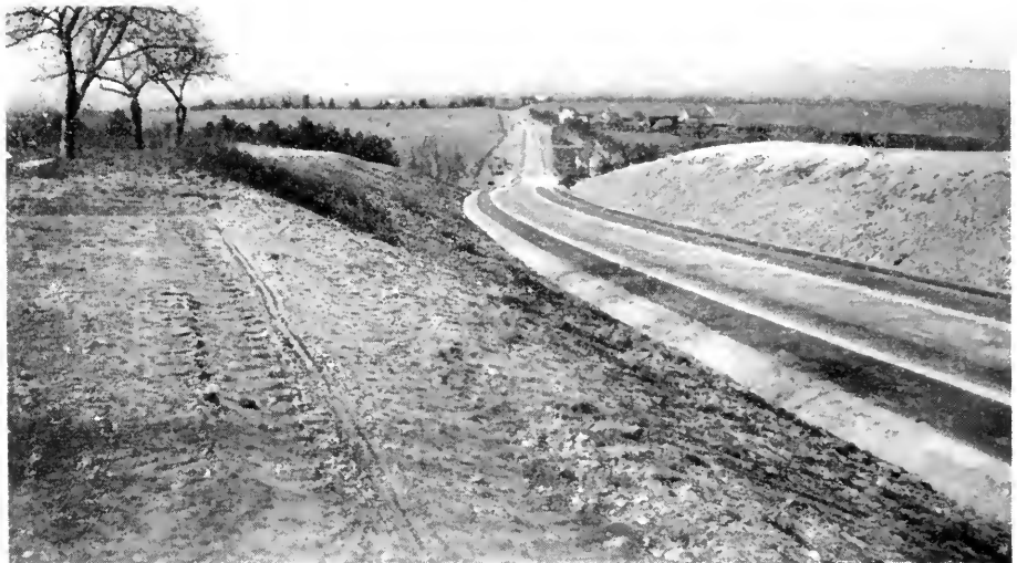
LOOKING EAST AND WEST RESPECTIVELY ACROSS THE NEW BRIDGE WHICH REPLACES THE OLD JUG BRIDGE OVER THE MONOCACY RIVER ON ROUTE 40
