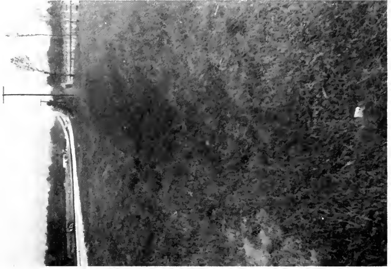
EROSION IS EASILY CONTROLLED IN WELL-ROUNDED GUTTERS. THE LEFT PICTURE SHOWS A HIGHLY EROSION GUTTER CONDITION WHICH WAS REMEDIED BY STREAMLINING AND SODDING AS SHOWN ON THE RIGHT
