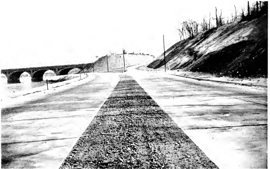
WATERVIEW AVENUE APPROACHING FROM THE OLD ANNAPOLIS ROAD, THE INTERCHANGE AT HANOVER STREET, CONSTRUCTED AS AN ACCESS HIGHWAY PROJECT IN BALTIMORE CITY
