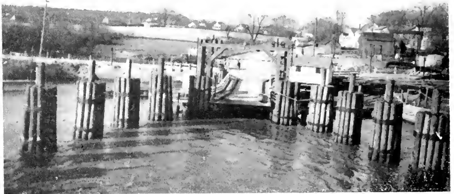
SOUTH APPROACH TO C. & D. CANAL FERRY
