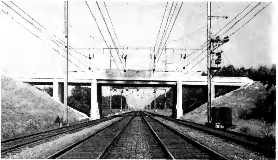
STEEL AND CONCRETE BRIDGE OVER PENNSYLVANIA RAILROAD ON MILITARY ACCESS ROAD FROM EDGEWOOD ARSENAL TO U. S. ROUTE 40, HARFORD COUNTY
