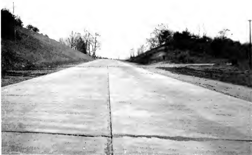
APPROACHING THE SANDY POINT TERMINAL OF THE SANDY POINT-MATAPEAKE FERRY
