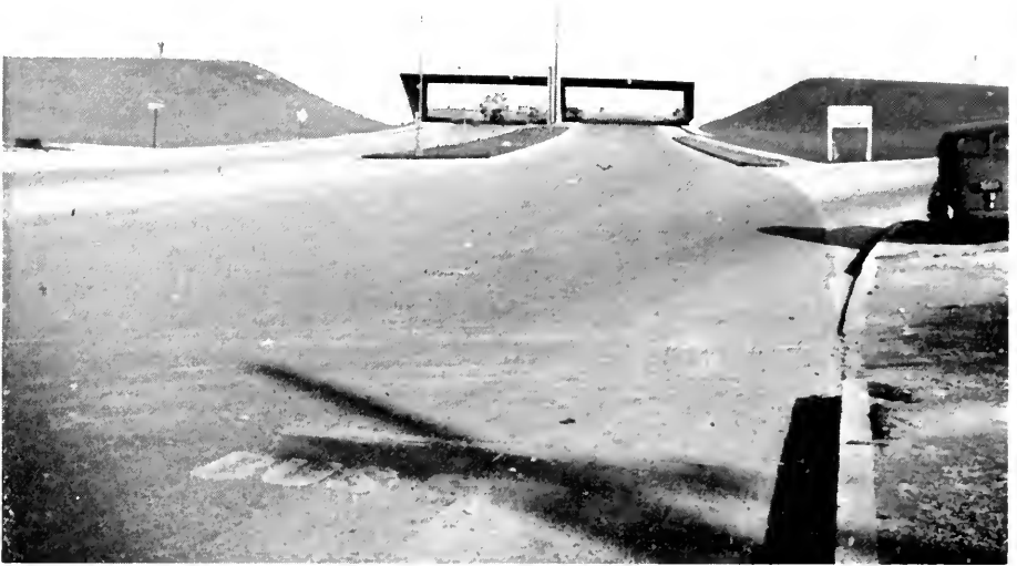
GRADE SEPARATION STRUCTURE AT THE INTERSECTION OF PHILADELPHIA ROAD, U. S. ROUTE 40, AND ERDMAN AVENUE—A PART OF THE CLOVERLEAF BUILT AS AN ACCESS HIGHWAY PROJECT IN BALTIMORE CITY
