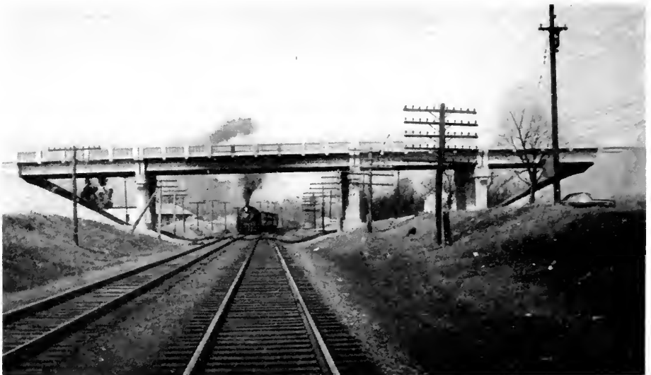
BRIDGE OVER BALTIMORE AND OHIO RAILROAD ON NEW MILITARY ACCESS ROAD FROM U. S. 81 AT LAUREL TO FORT GEORGE G. MEADE
