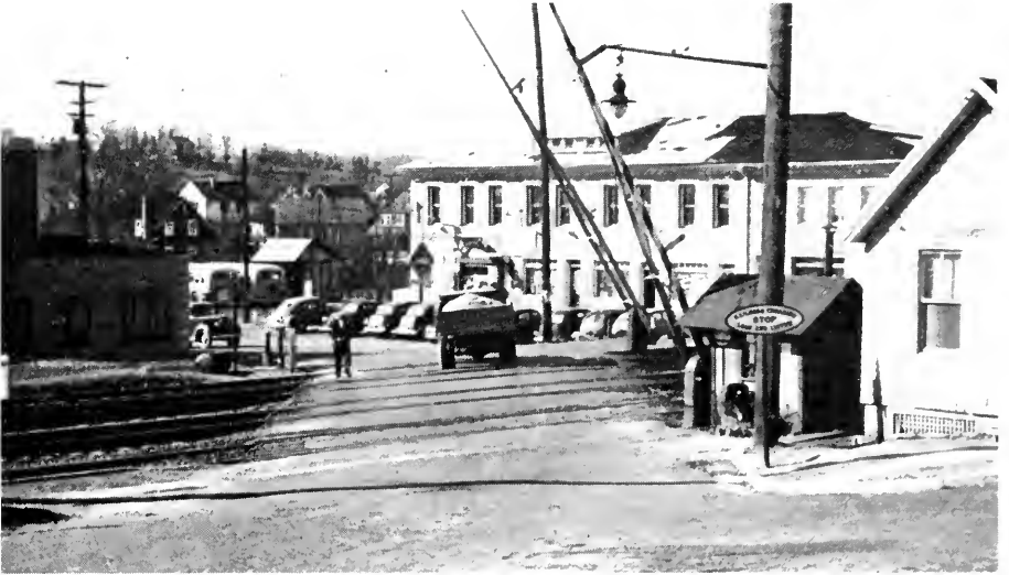
FRANCIS AVENUE CROSSING OF PENNSYLVANIA RAILROAD AT HALETHORPE
