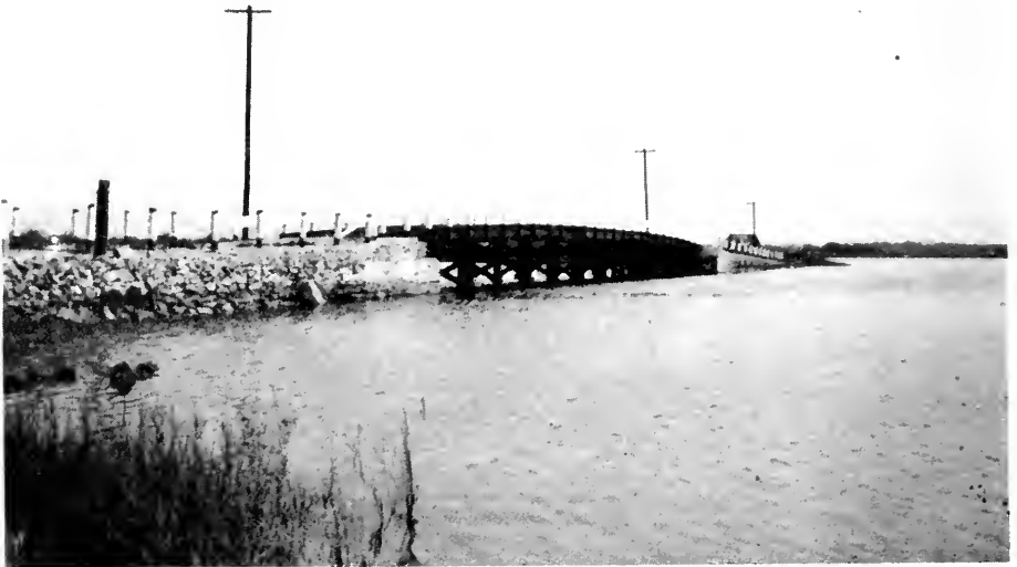
EASTERN NECK ISLAND BRIDGE BETWEEN KENT COUNTY MAINLAND AND EASTERN NECK ISLAND—AFTER REBUILDING
