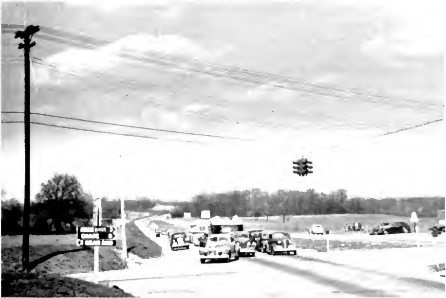
TAIL END OF WORK SHIFT. EFFECT OF HIGHWAY INTERSECTION AT GRADE. GOLDEN RING ROAD AND U. S. ROUTE 40
