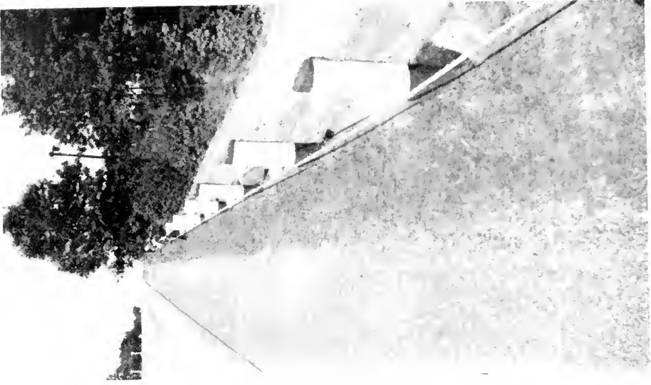
LEFT SHOWS THE EFFECT OF ROADSIDE EROSION ON THE GUARD RAIL. RIGHT, A WINDROW OF SOD PLACED AT THE GUARD RAIL TO INTERCEPT WATER AND PERMIT RUN-OFF, AT DESIGNATED INTERVALS OVER SOD FLUMES HAS BEEN FOUND TO BE VERY EFFECTIVE IN STABILIZING GUARD RAILS
