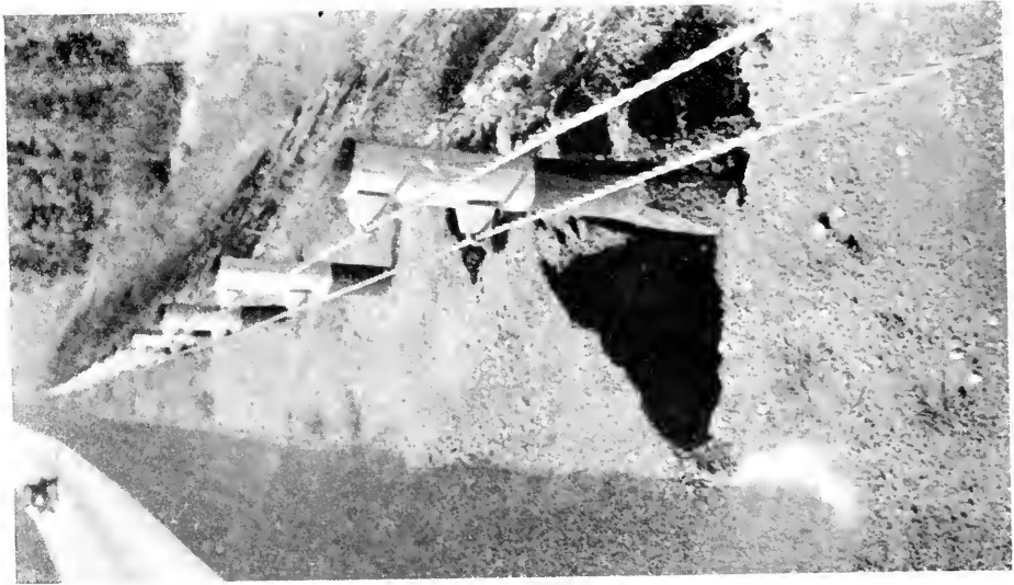
LEFT SHOWS THE EFFECT OF ROADSIDE EROSION ON THE GUARD RAIL. RIGHT, A WINDROW OF SOD PLACED AT THE GUARD RAIL TO INTERCEPT WATER AND PERMIT RUN-OFF, AT DESIGNATED INTERVALS OVER SOD FLUMES HAS BEEN FOUND TO BE VERY EFFECTIVE IN STABILIZING GUARD RAILS
