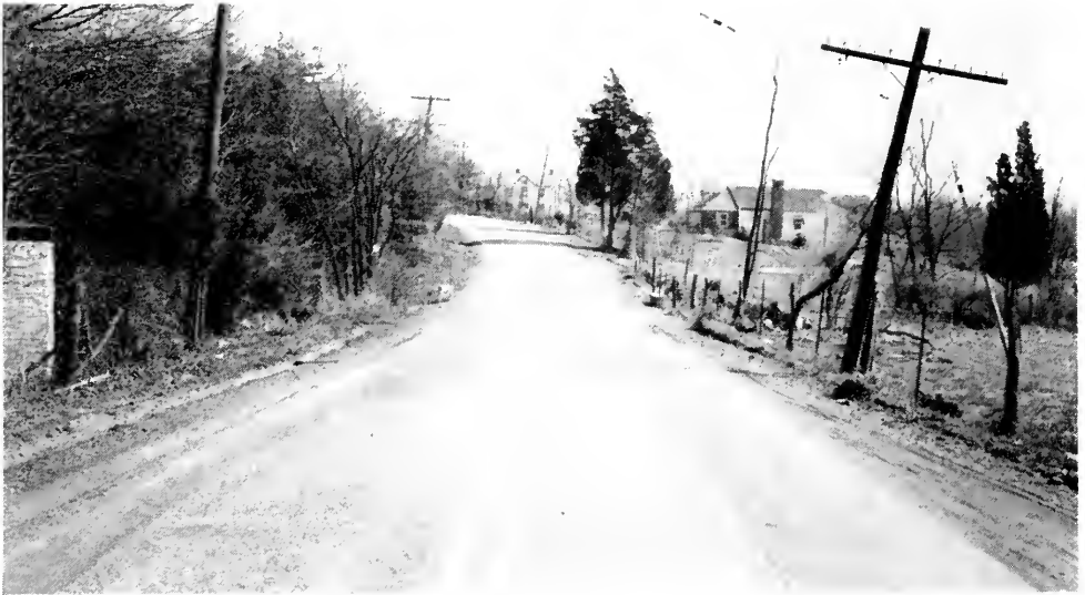
SECTION OF MD. ROUTE 28 NEAR DARNESTOWN, MD. BEFORE WIDENING AND RESURFACING
