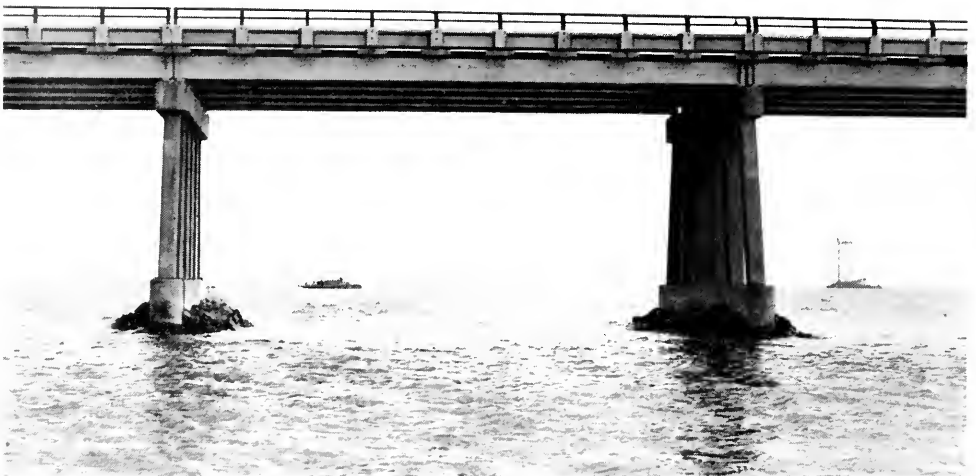
STONE PROTECTION AROUND WEST BENTS—CHESAPEAKE BAY BRIDGE
