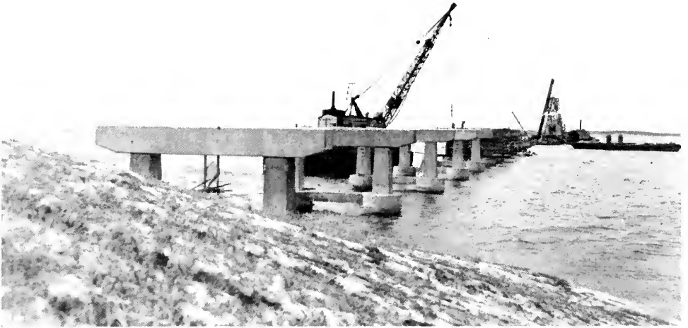
CONSTRUCTION OF EAST BENTS—CHESAPEAKE BAY BRIDGE
