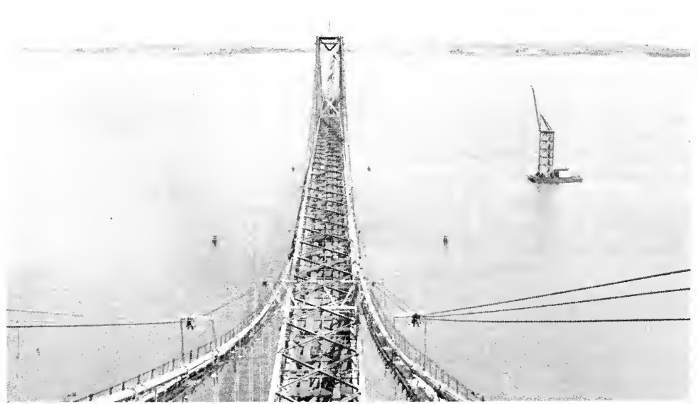
MAIN SPAN SUSPENSION BRIDGE—CHESAPEAKE BAY BRIDGE
