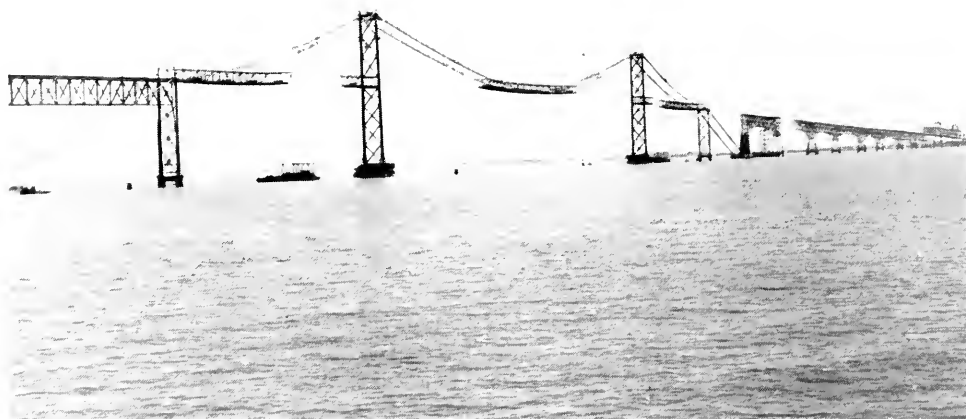
ERECTING OF SUSPENSION BRIDGE TRUSSES—CHESAPEAKE BAY BRIDGE
