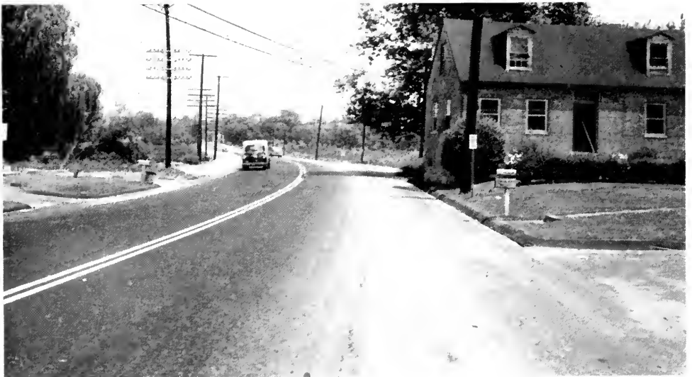
SAME LOCATION AFTER IMPROVEMENT—WORK PERFORMED BY PRISON LABOR
