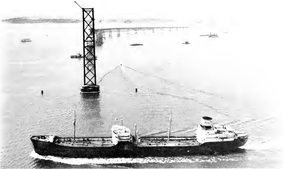
MAIN SAILING SPAN—CHESAPEAKE BAY BRIDGE
