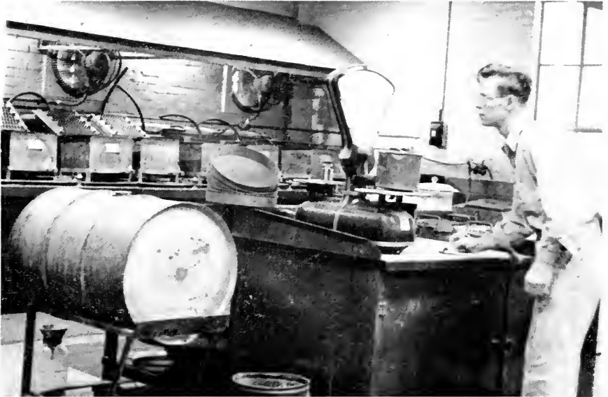
RECORDING WEIGHT OF AGGREGATE—BITUMINOUS CONCRETE EXTRACTION PROCESS
