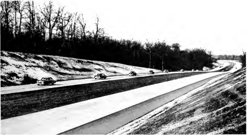
RELOCATED DIVIDED HIGHWAY WITH CONTROL OF ACCESS FEATURES—BALTIMORE NATIONAL PIKE BETWEEN WEST FRIENDSHIP AND MORGAN STATION
