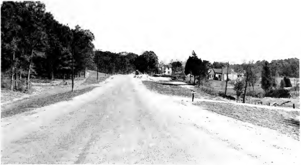
SAME LOCATION AFTER IMPROVEMENT—SHOWING RELOCATION—WORK PERFORMED BY PRISON LABOR
