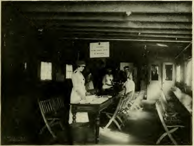
READING ROOM IN SWITCH YARD CANTEN
