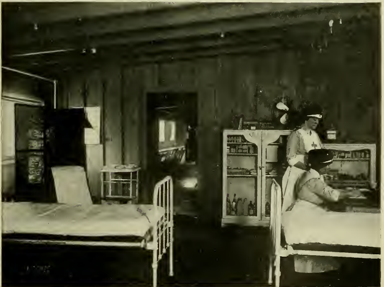
EMERGENCY ROOM IN SWITCH YARD CANTEN
