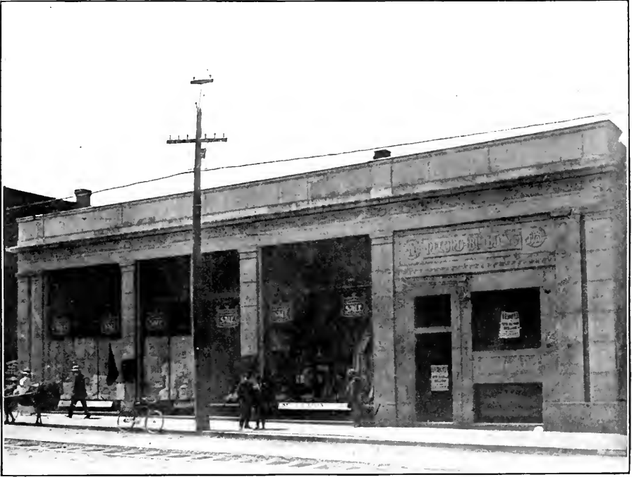
Halifax granite. Record building, Sydney, N.S.
