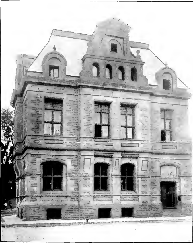
Miramichi sandstone. Post-office, Newcastle, N.B.
