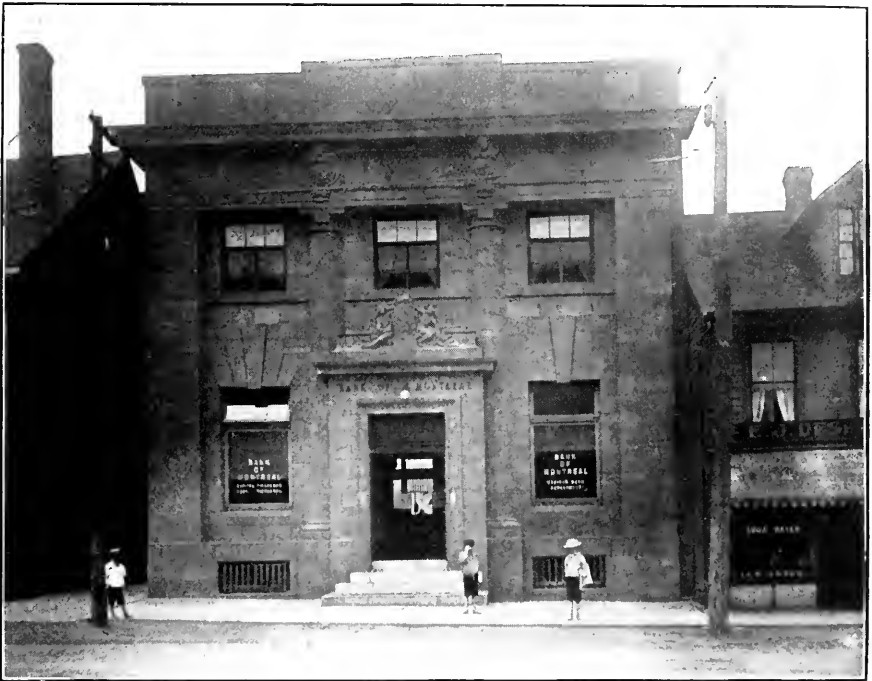
Prince Edward Island sandstone. Bank of Montreal, Charlottetown, P.E.I.
