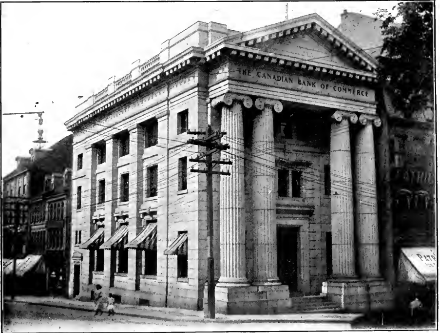
Terence Bay granite. Bank of Commerce, Halifax, N.S.
