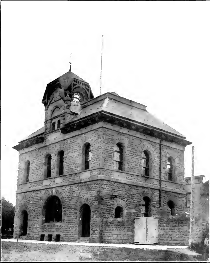
Grande Anse sandstone. Post-office, Bathurst, N.B.
