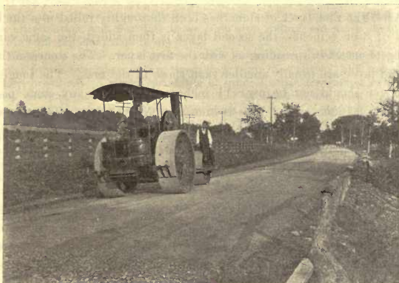
FIG. 15.—Rolling surface of macadam road on state highway in Massachusetts.
