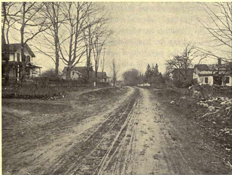
FIG. 33.—Gravel road in southwestern Connecticut.
