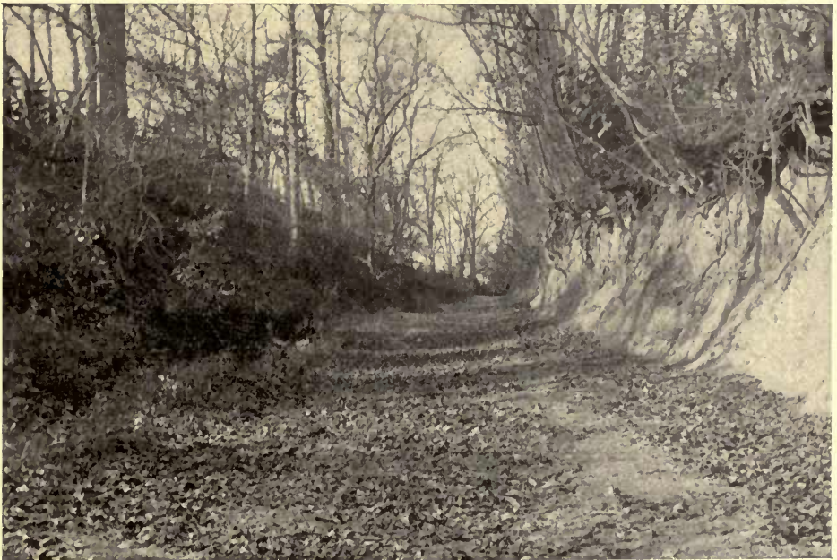
FIG. 2.—UNDRAINED ROAD IN CUT, CHARLES COUNTY.
