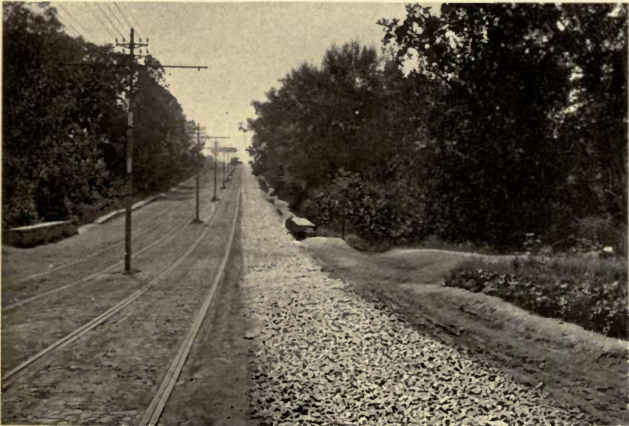
FIG. 2.—GNEISS ROAD, BALTIMORE CITY. STONE SPREAD WITHOUT ROLLING.
