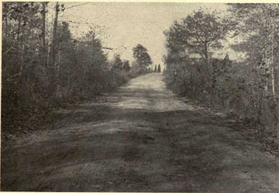
FIG. 1.—GRAVEL ROAD, PRINCE GEORGE'S COUNTY.
