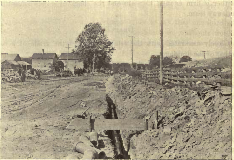
FIG. 7.—Laying side-drain for macadam road on state highway in Massachusetts.
