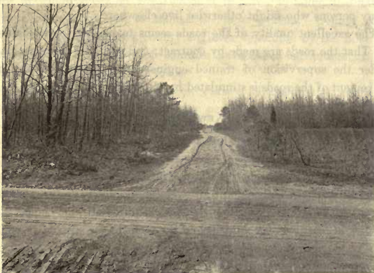
FIG. 35.—Sandy road with improved gravel road in foreground, New Jersey.
