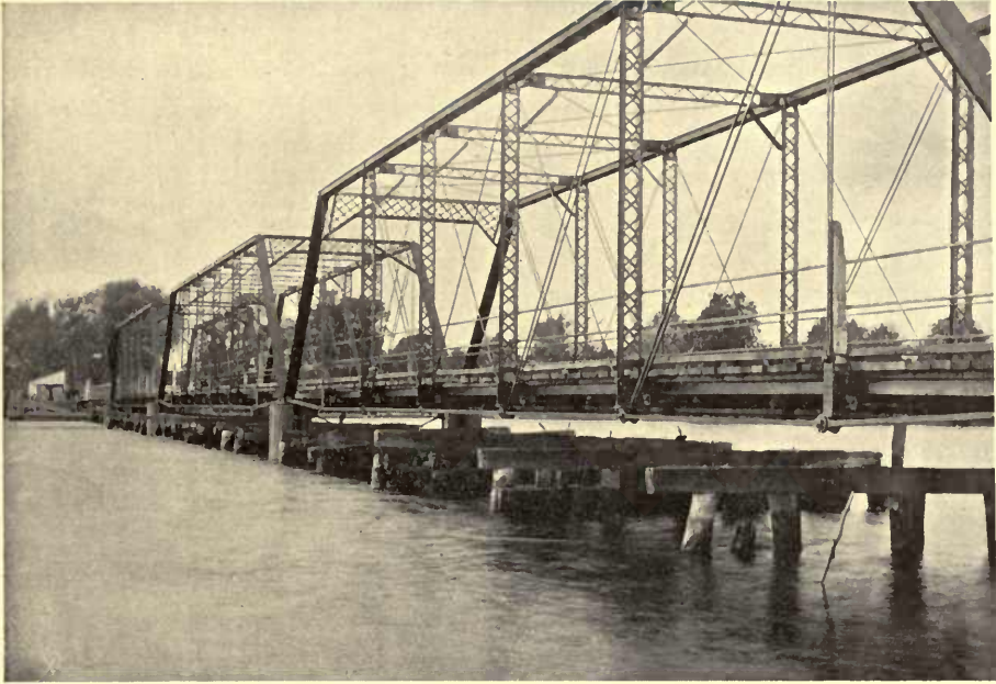
FIG. 1.—IRON BRIDGE OVER CHOPTANK RIVER, CAROLINE COUNTY.
