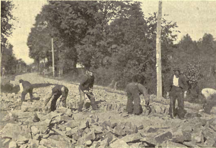
FIG. 16.—Laying telford road on state highway in Massachusetts.
