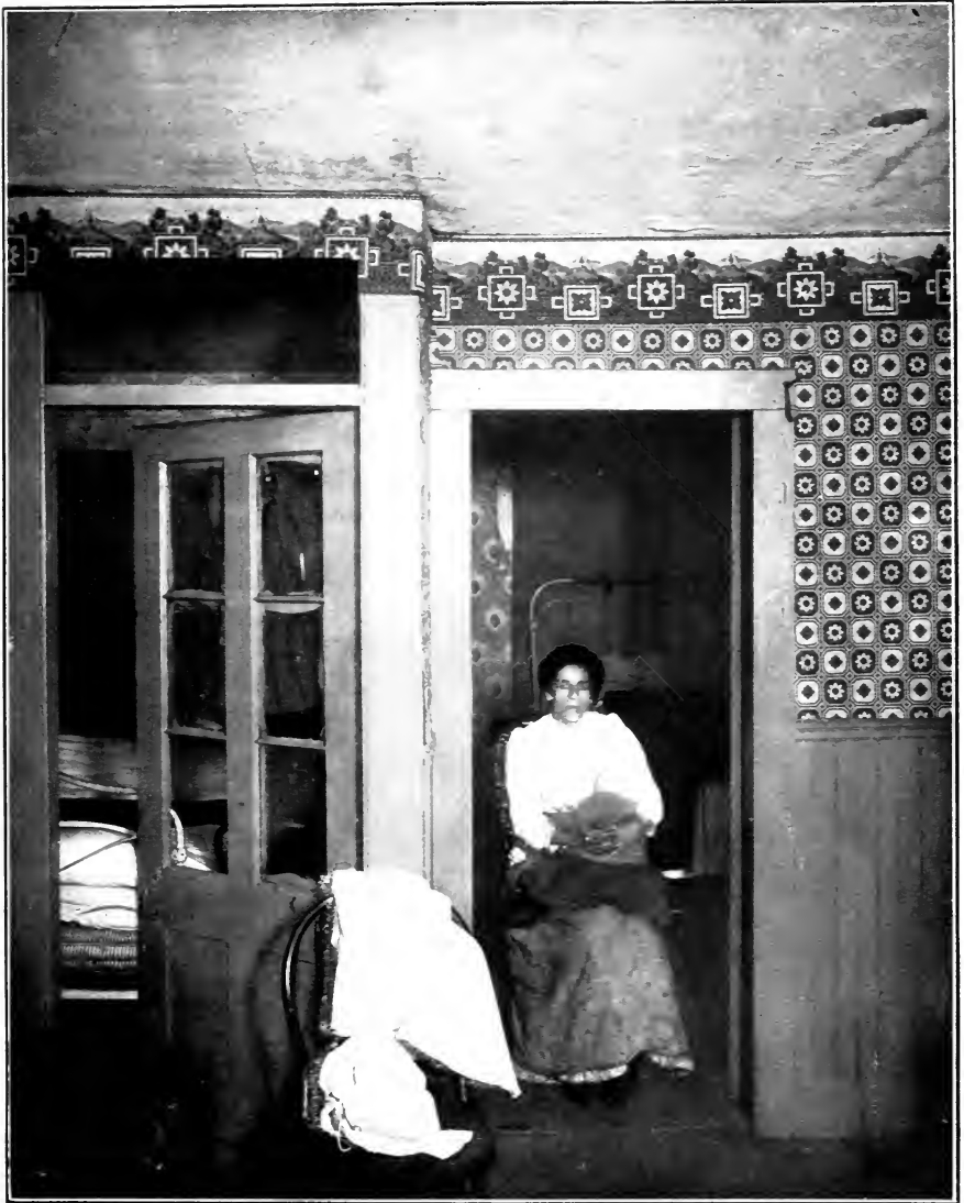
This shows two dark bedrooms opening from a very gloomy kitchen—one bedroom has a window about 24 x 30 opening into a poorly ventilated hall. The bedroom on the right has a window (full size) opening outside, but the adjoining building is so near that very little light enters here. The same is true of the kitchen. This tenement is cold and damp.
