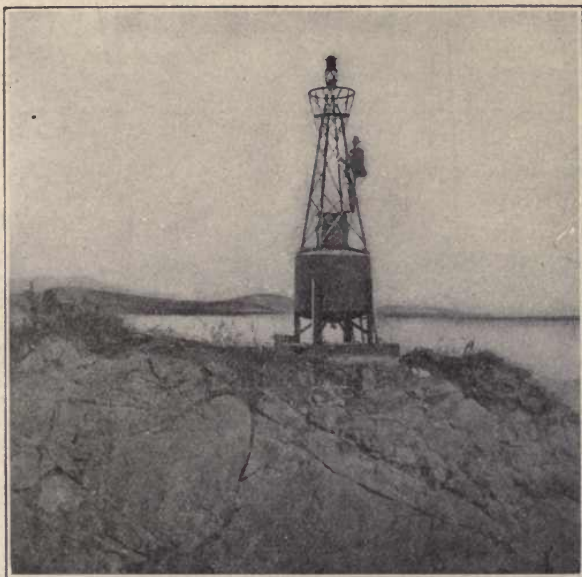
Dock Island, British Columbia, light, on the run between Victoria and Vancouver, installed March 7, 1906. It contains a 200 mm. lantern, is charged with 1,000 pounds of carbide, and runs four months without recharging. As will be seen, no particular care is taken with regard to temperature conditions.
