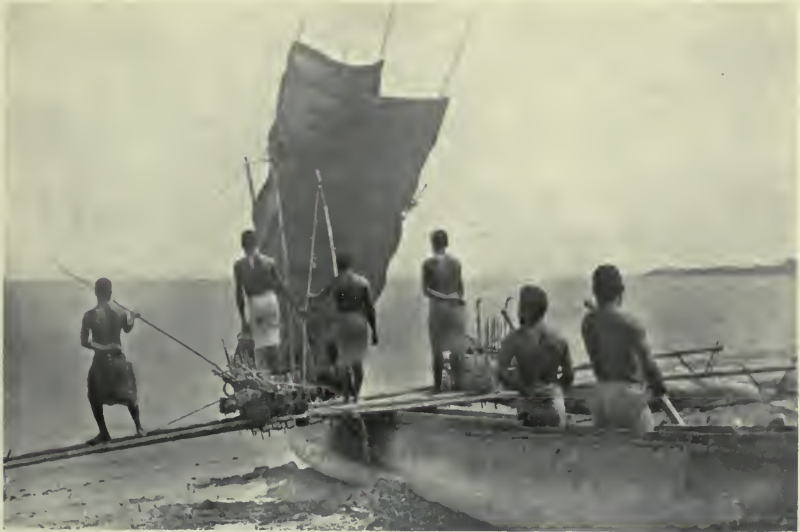
FIG. 1. Midships view of a Mabuiag canoe with mat sails, 1888 (pp. 205, 207—213).
