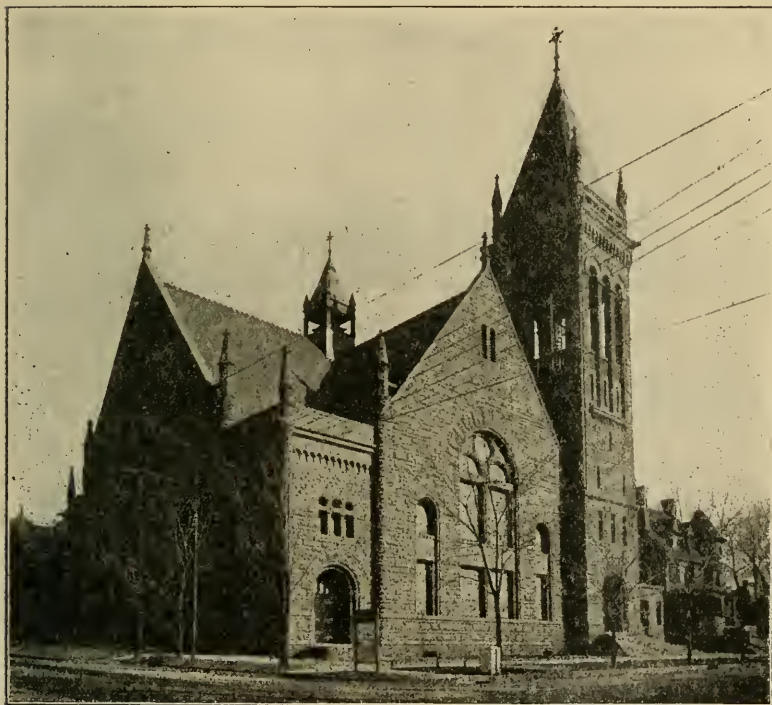
CENTRAL PRESBYTERIAN CHURCH, DENVER, COLO.
