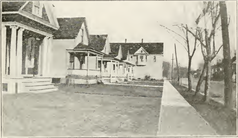
Property values destroyed by the projection of a building beyond the natural building line.
