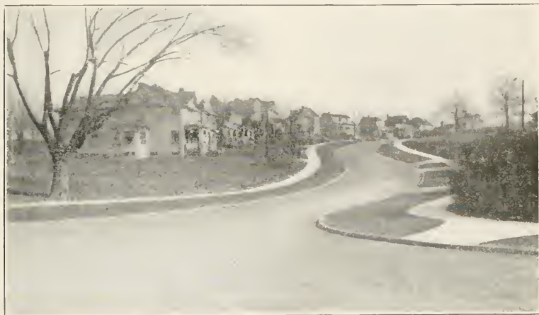
HILLCREST AVE., McCLELLAN HEIGHTS An example of a street well laid out to fit rough topography.
