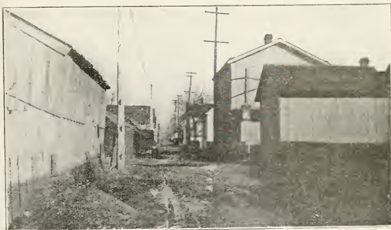
House facing alley in West Davenport.
