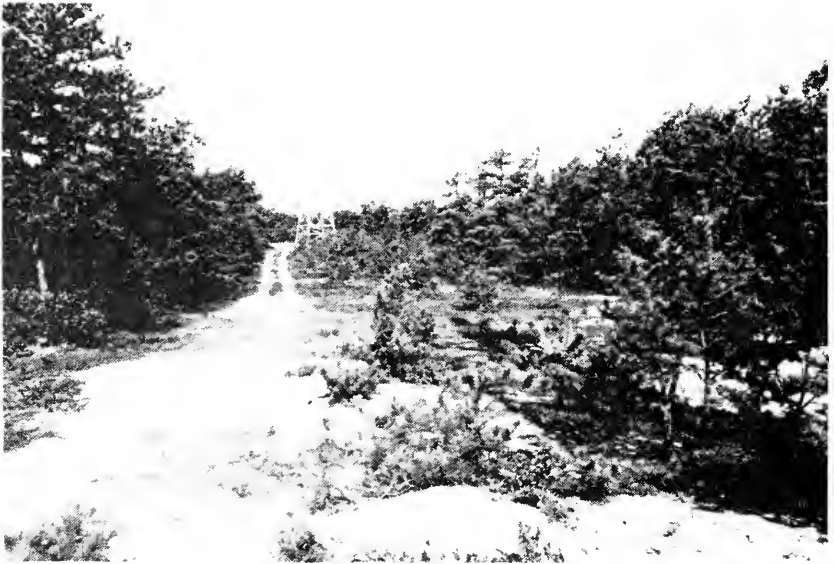
Figure 1b. At completion of right-of-way. a
