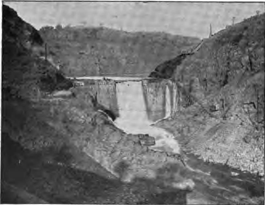
FIG. 86.—LA GRANGE DAM, CALIFORNIA.
