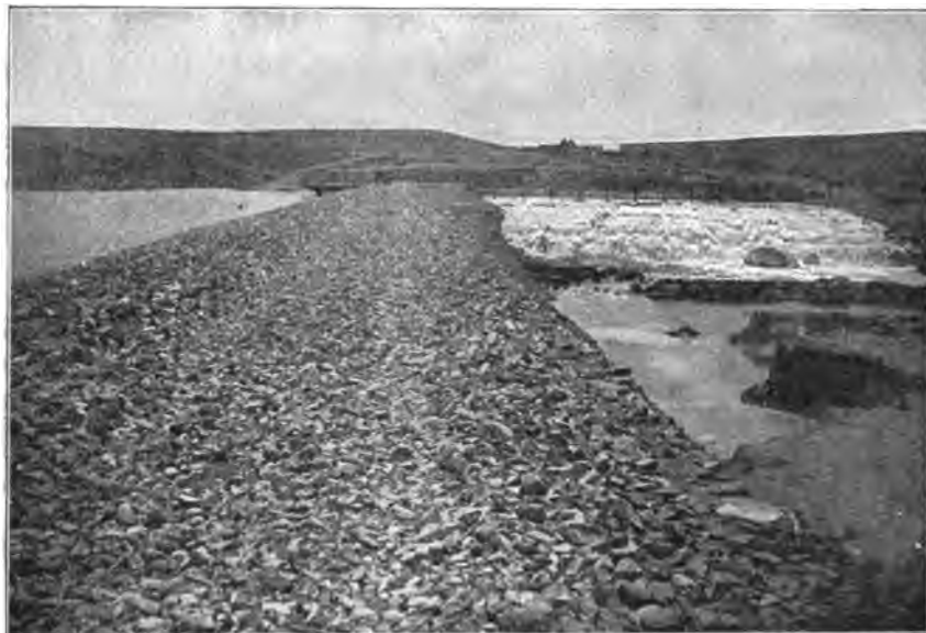
FIG. 27.—LAKE AVALON DAM, PECOS RIVER, NEW MEXICO. SHOWING THE CREST OF COMPLETED DAM AND SPILLWAY DISCHARGING.
