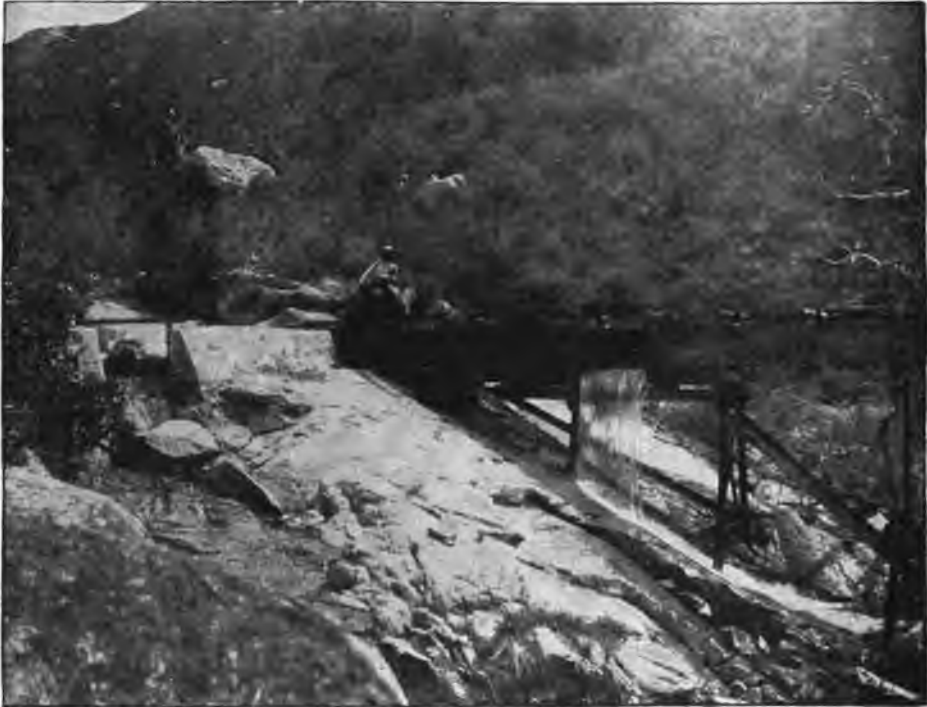
FIG. 8.—PICK-UP WEIR AT HEAD OF DISTRIBUTING SYSTEM IN ESCONDIDO IRRIGATION DISTRICT.
