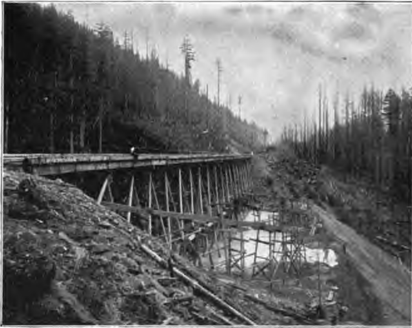
FIG. 52.—NORTHERN PACIFIC RAILWAY. BRIDGE 190.
