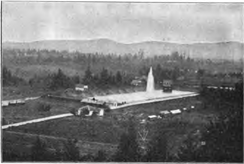
FIG. 121.—RESERVOIR No. 2, PORTLAND, OREGON, SHOWING AERATING FOUNTAIN 125 FEET HIGH.
