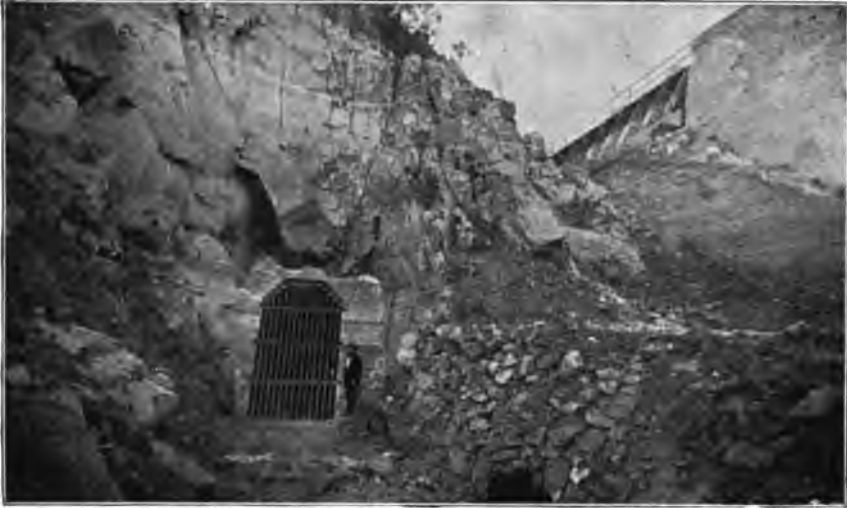
FIG. 70.—SWEETWATER DAM, SHOWING HEAD OF OUTLET TUNNEL AND SPILLWAY.
