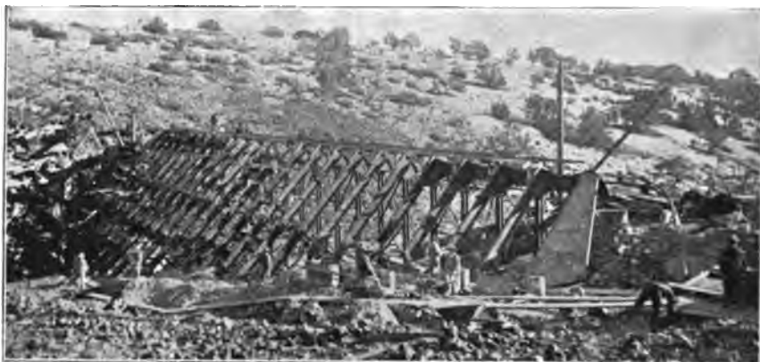
FIG. 113.—ASH FORK, STEEL DAM, SHOWING FRAME READY TO RECEIVE PLATES.
