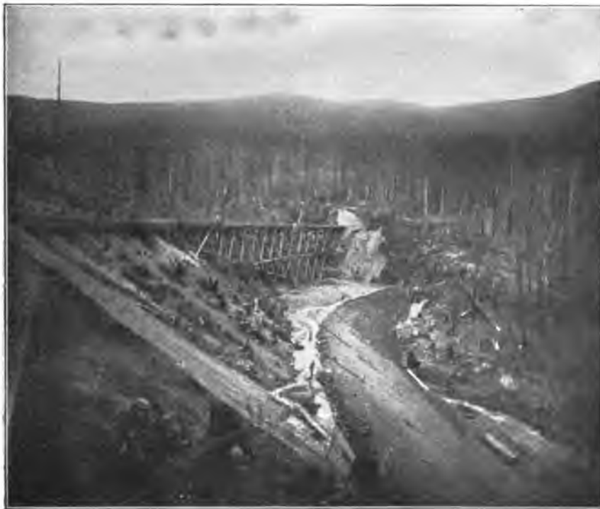
FIG. 55.—NORTHERN PACIFIC RAILWAY, BRIDGE 184. HYDRAULIC FILLING IN PROGRESS.
