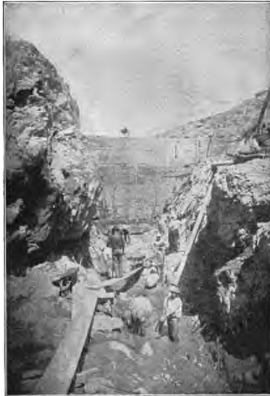
FIG. 11 — MASONRY FOUNDATION OF LOWER OTAY DAM.
