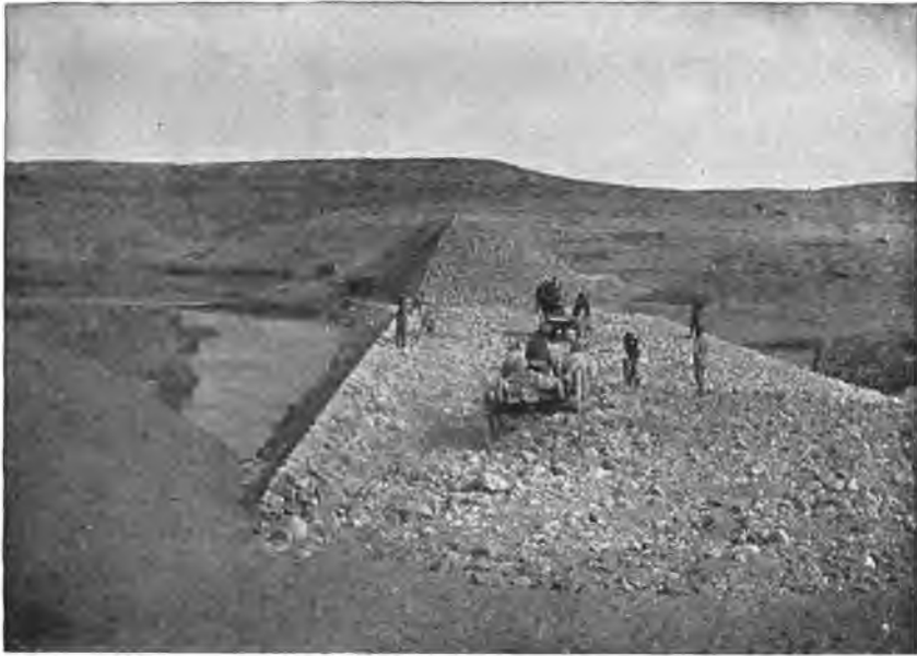
FIG. 26.—LAKE AVALON DAM. ROCK-FILL IN PROCESS OF CONSTRUCTION.
