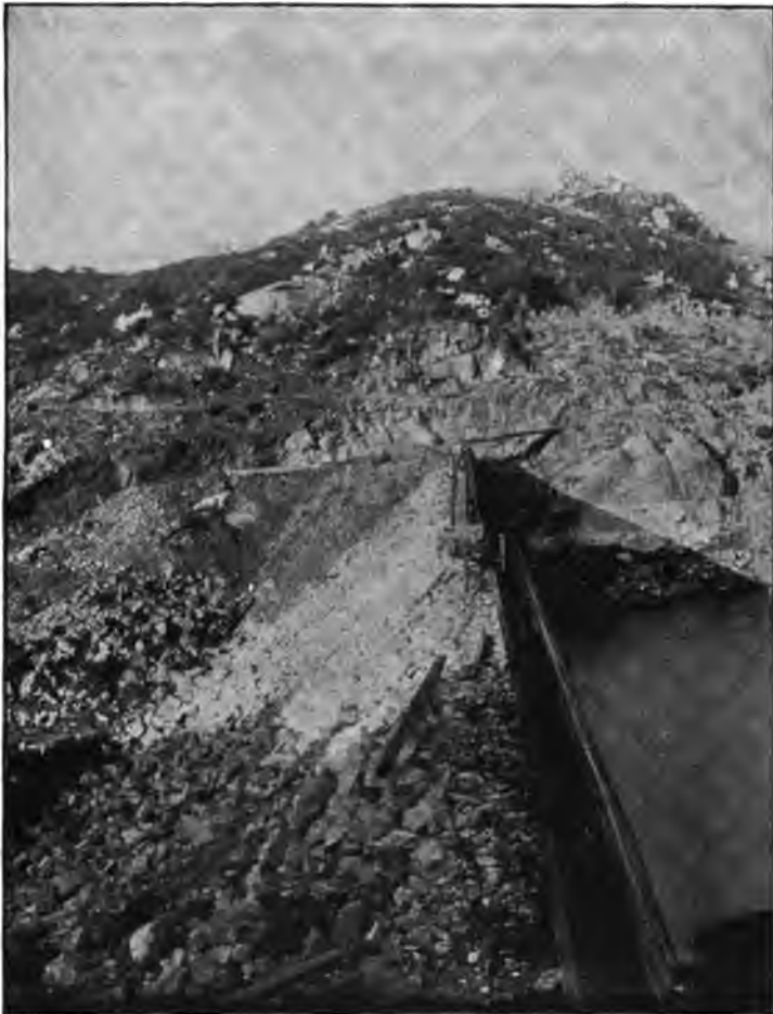
FIG. 4.—ESCONDIDO IRRIGATION DAM, LOOKING NORTH, SHOWING SPILLWAY.
