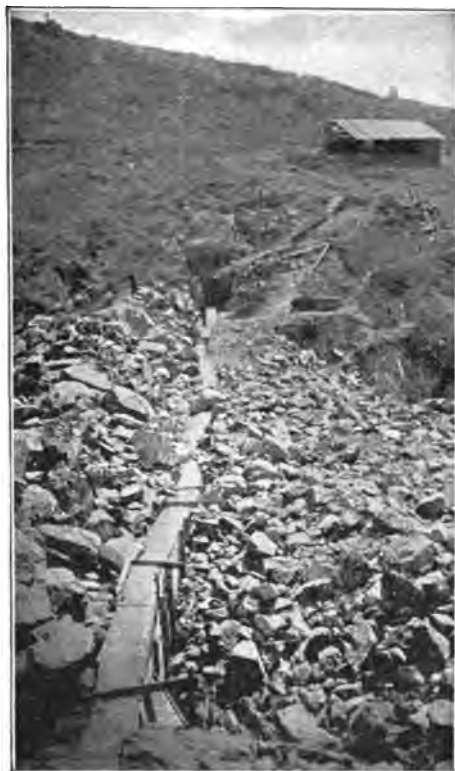
FIG. 13.—CREST OF LOWER OTAY DAM, SHOWING WEB-PLATE OF STEEL EMBEDDED IN CONCRETE. DAM NEARING COMPLETION.
