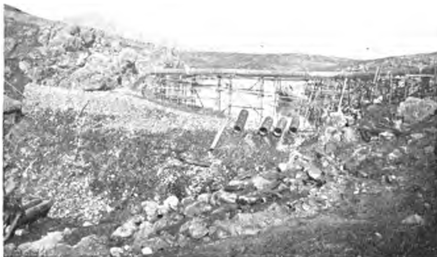
FIG. 48.—LA MESA HYDRAULIC-FILL DAM, SHOWING PIPE DISCHARGING MATERIAL ON THE DAM.
