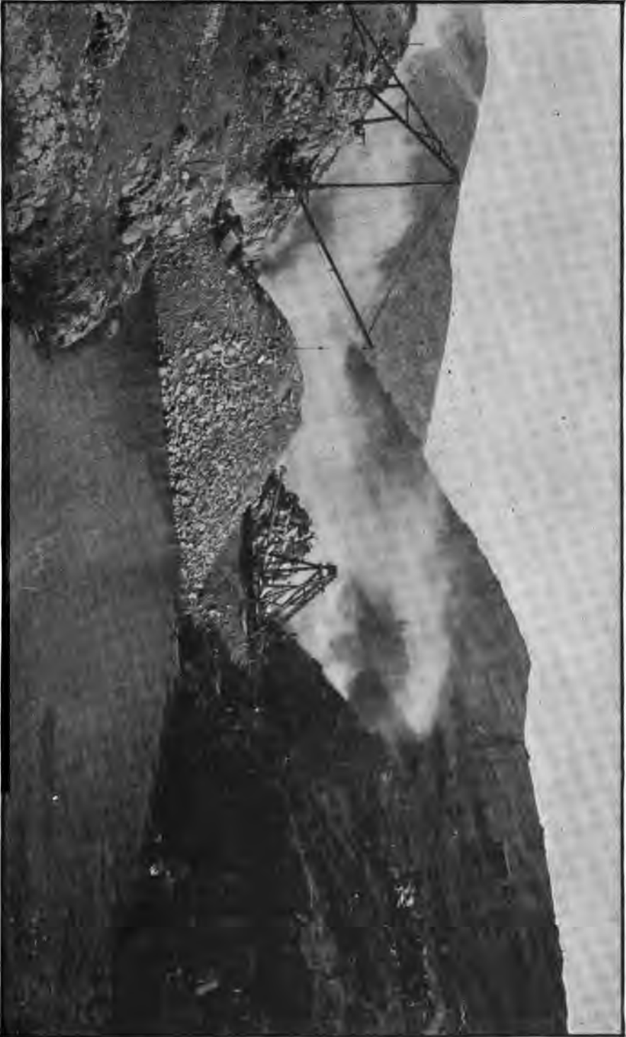
FIG. 16.—EXPLOSION OF GREAT BLAST AT LOWER OTAY ROCK FILL DAM.
