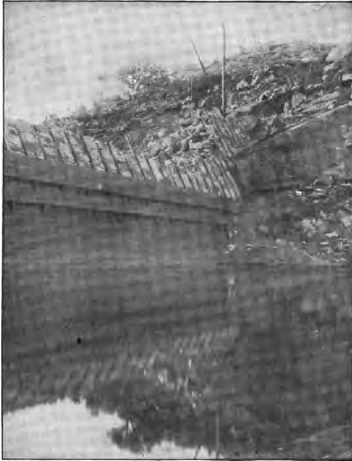
FIG. 10.—CONSTRUCTION OF FACING OF ESCCONDIDO DAM.
