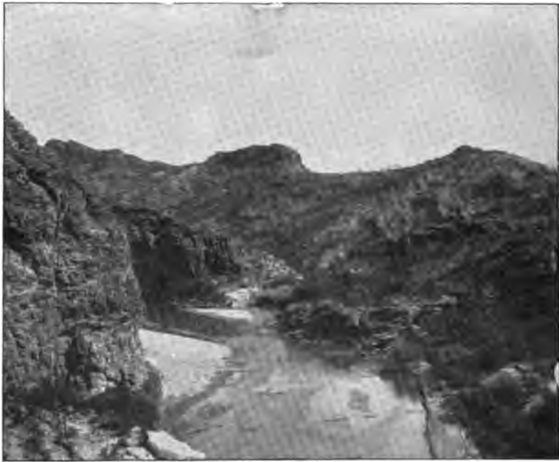
FIG. 155a.—BUTTES DAM-SITE, LOOKING UP-STREAM FROM UPPER TOE.
