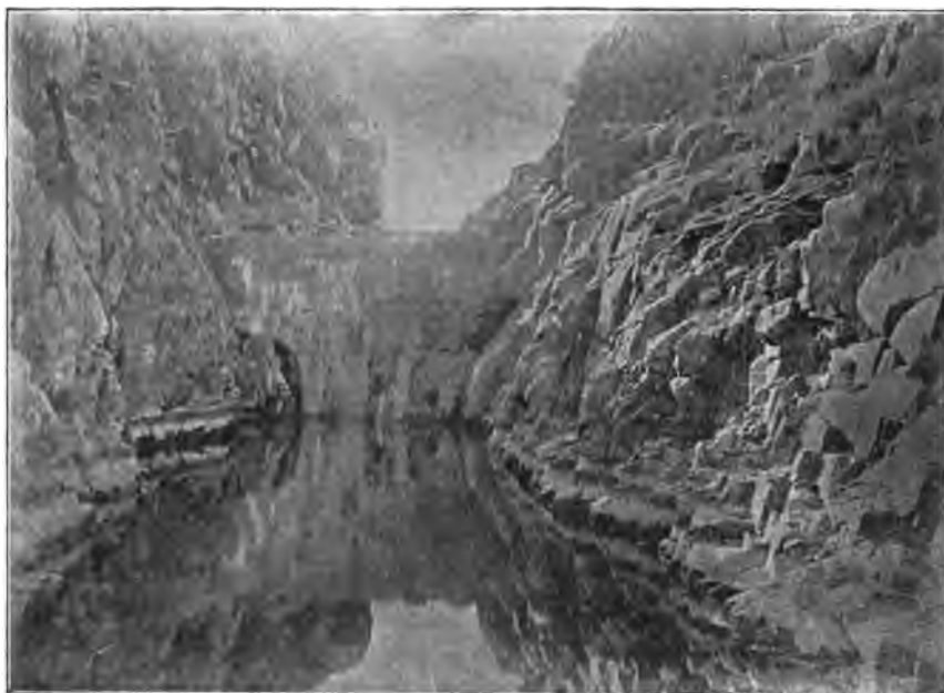
FIG. 22.—UPPER OTAY DAM, FOUNDATION MASONRY.
