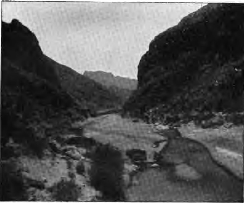
FIG. 152a.—SAN CARLOS DAM-SITE, LOOKING DOWN-STREAM.
