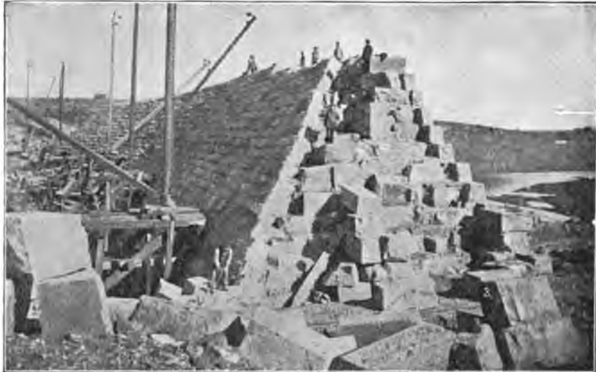
FIG. 109.—SELIGMAN DAM, ARIZONA.
