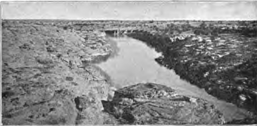
FIG. 114.—ASH FORK RESERVOIR.
