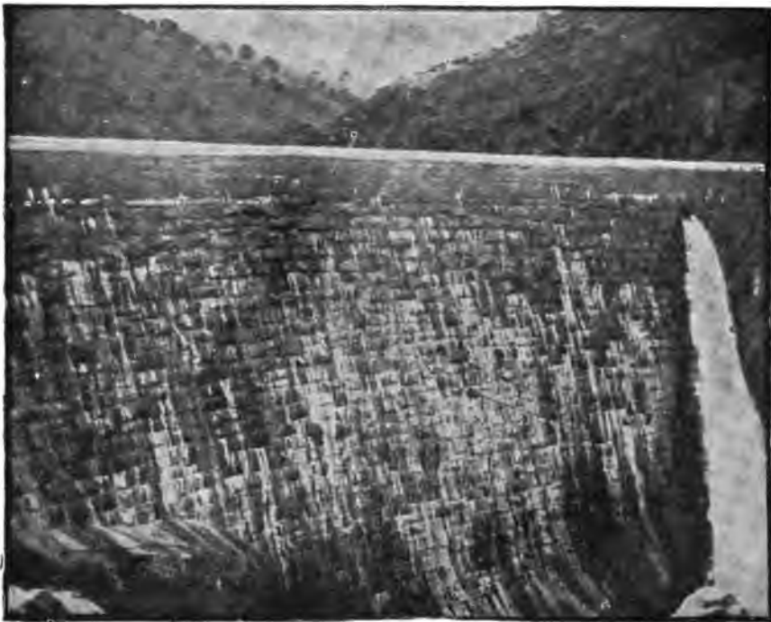
FIG. 84.—LOWER FACE OF LA GRANGE DAM.
