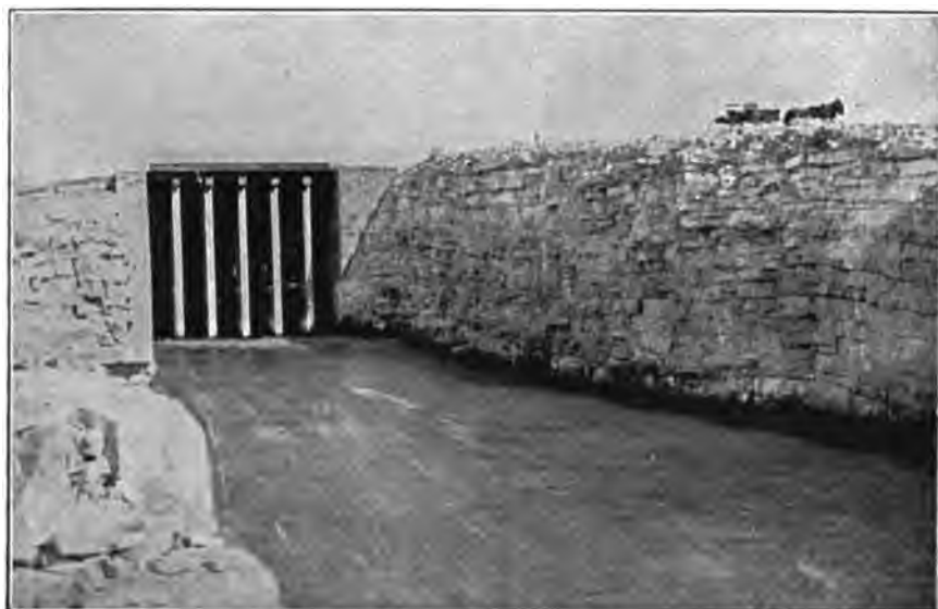
FIG. 28.—CANAL HEADGATES, LAKE AVALON DAM.
