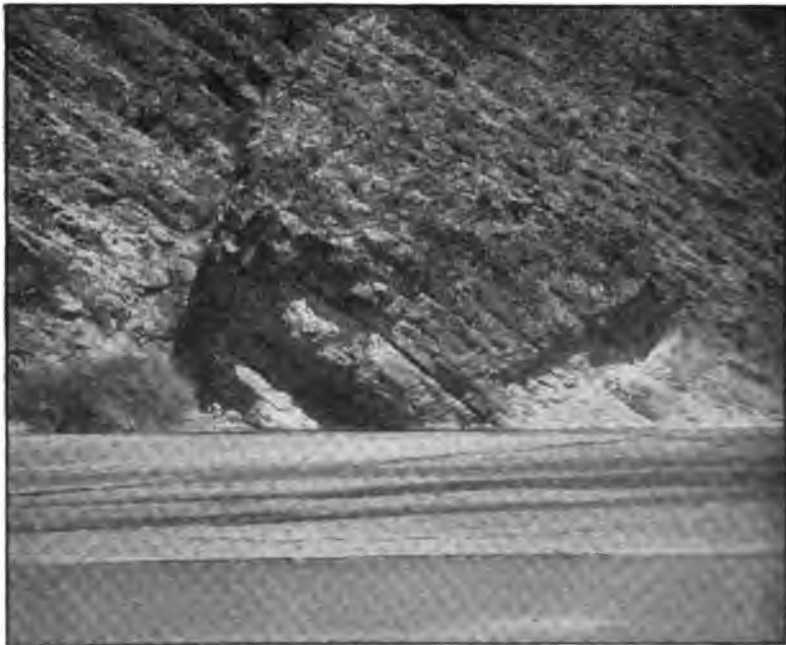
FIG. 154a.—VIEW OF LEFT ABUTMENT WALL, SAN CARLOS DAM-SITE, SHOWING DIP OF LIMESTONE.
