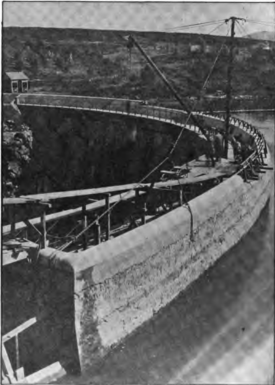
FIG. 66.—REPAIRING AND INCREASING THE HEIGHT OF THE PARAPET OF SWEET-WATER DAM.
