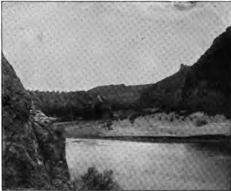
FIG. 156.—BUTTES DAM-SITE, LOOKING UP-STREAM; PROPOSED QUARRIES ON LEFT; SPILLWAY ON LEFT OF CENTER OF FIELD.
