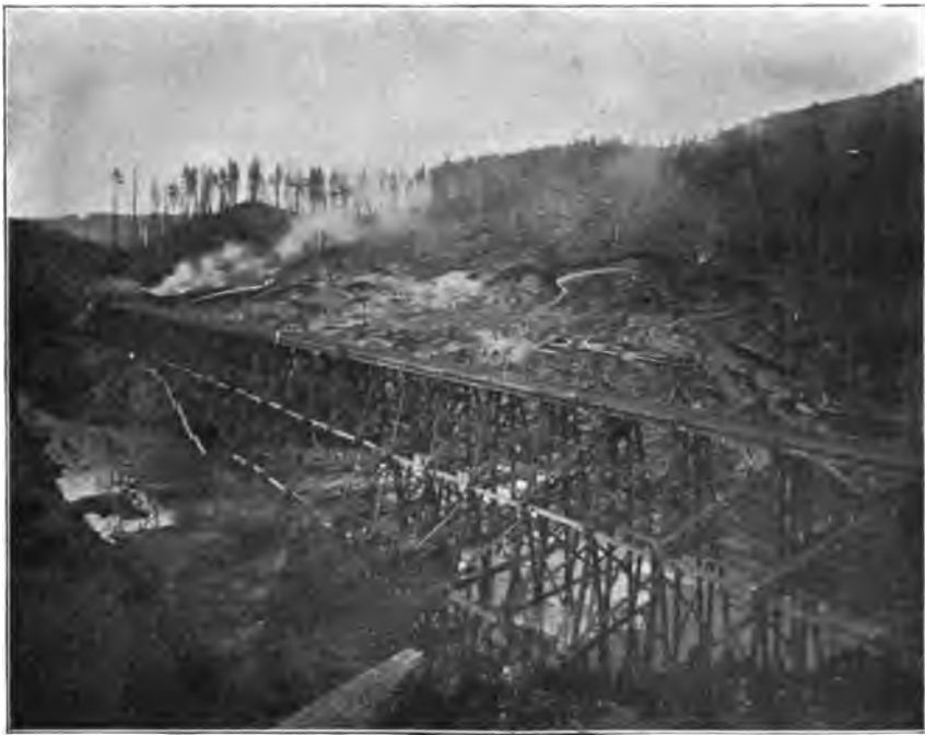
FIG. 53.—NORTHERN PACIFIC RAILWAY. BRIDGE 189, CASCADE MOUNTAINS.
