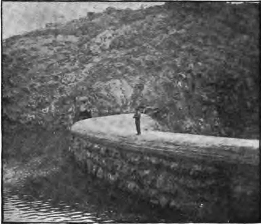
FIG. 88.—UPPER FACE OF LA GRANGE DAM.
