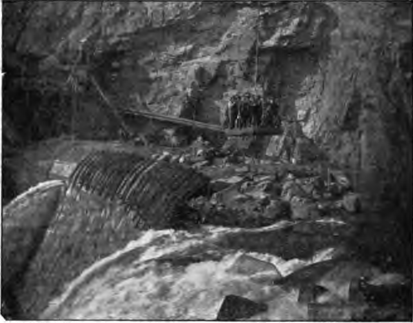
FIG. 85.—LA GRANGE DAM, CALIFORNIA, DURING CONSTRUCTION—FINISHING THE CREST.
