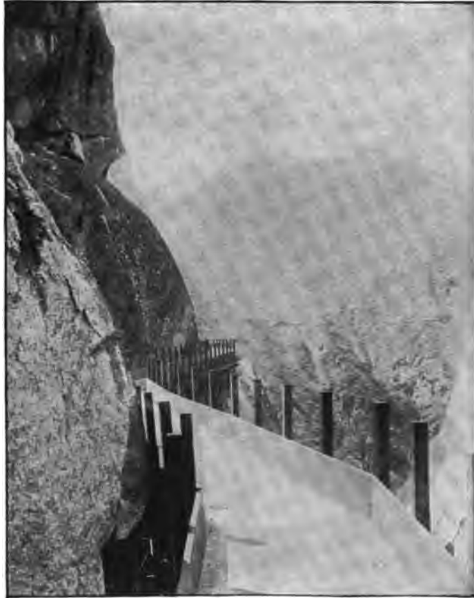
FIG. 3.—FEEDER CONDUIT OF ESCONDIDO IRRIGATION DISTRICT.
