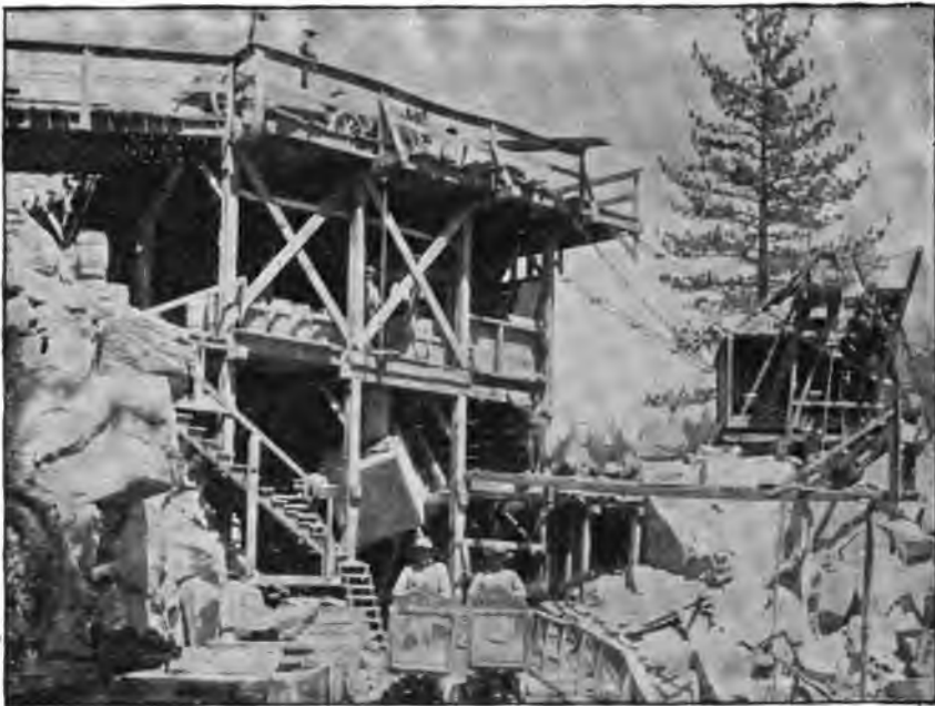
FIG. 76.—HEMET DAM CONSTRUCTION PLANT.
