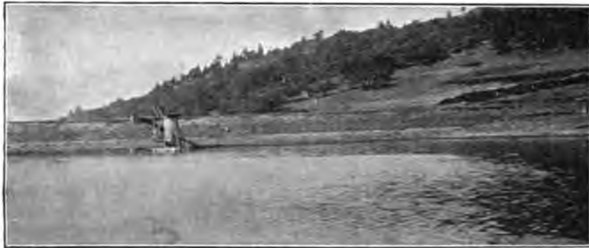
FIG. 128.—VIEW OF CUYAMACA DAM AND OUTLET-TOWER.
