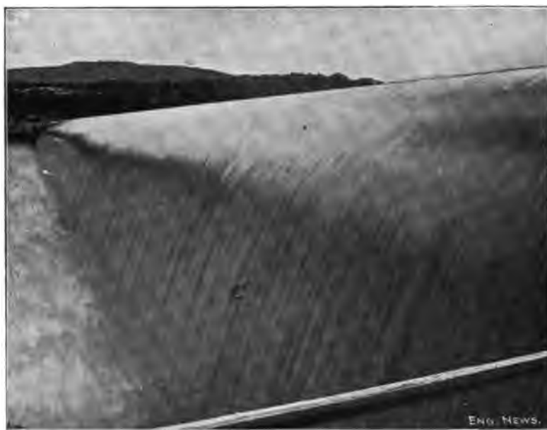
FIG. 123a.—AUSTIN DAM DURING FLOOD OF APRIL 7, 1900, AND IMMEDIATELY BEFORE THE BREAK.
