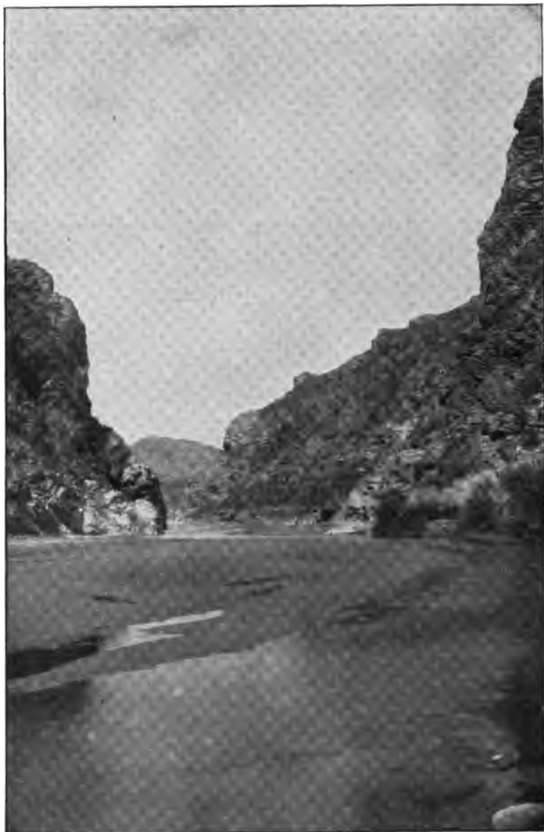
FIG. 154.—VIEW OF THE SAN CARLOS DAM-SITE, GILA RIVER, ARIZONA.
