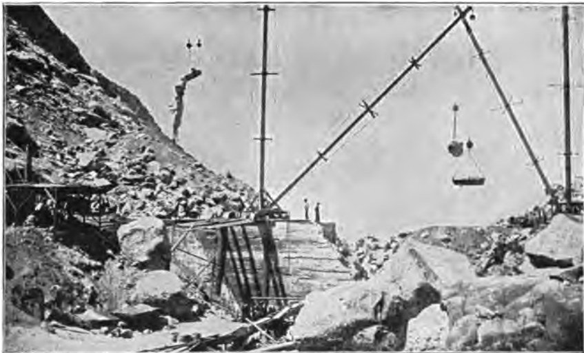
FIG. 20.—MORENA ROCK-FILL DAM, SHOWING A PORTION OF TOE-WALL UNDER CONSTRUCTION.
