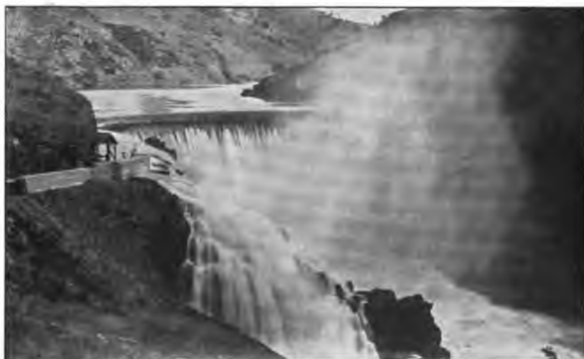
FIG. 88.—LA GRANGE DAM, CALIFORNIA, DURING FLOOD.
