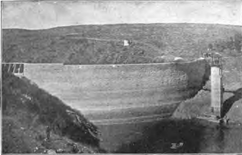
FIG. 60.—FACE OF SWEETWATER DAM IN 1899. AFTER TWO YEARS OF DROUTH.
