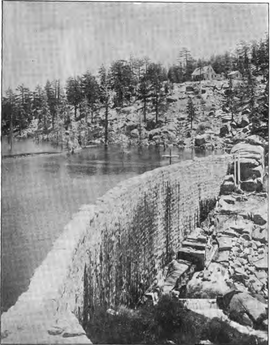
FIG. 79.—BEAR VALLEY DAM, LOOKING SOUTH, TOWARD SPILLWAY.
