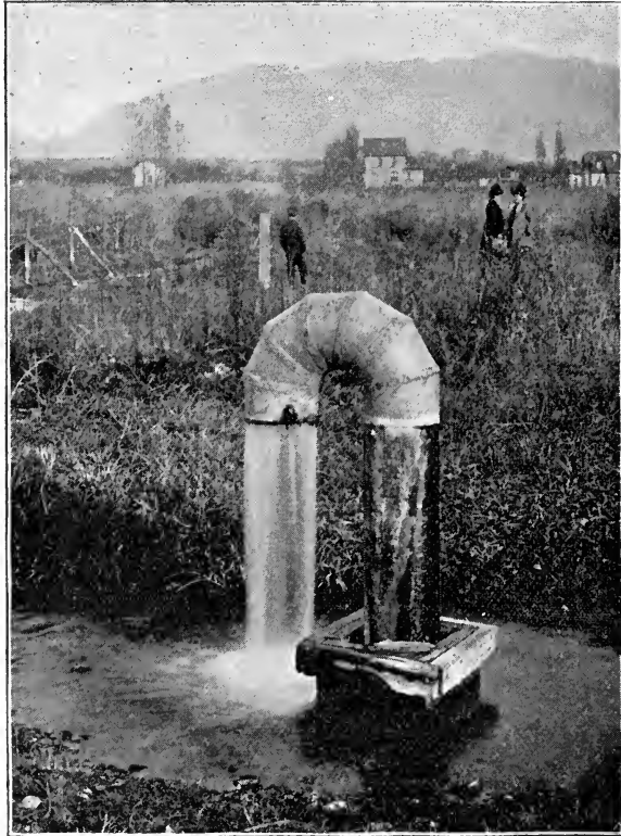
FLOWING WELL, NEAR SALT LAKE CITY.
