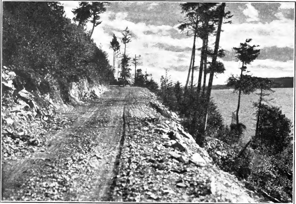
Along the Park-to-Park Highway.
