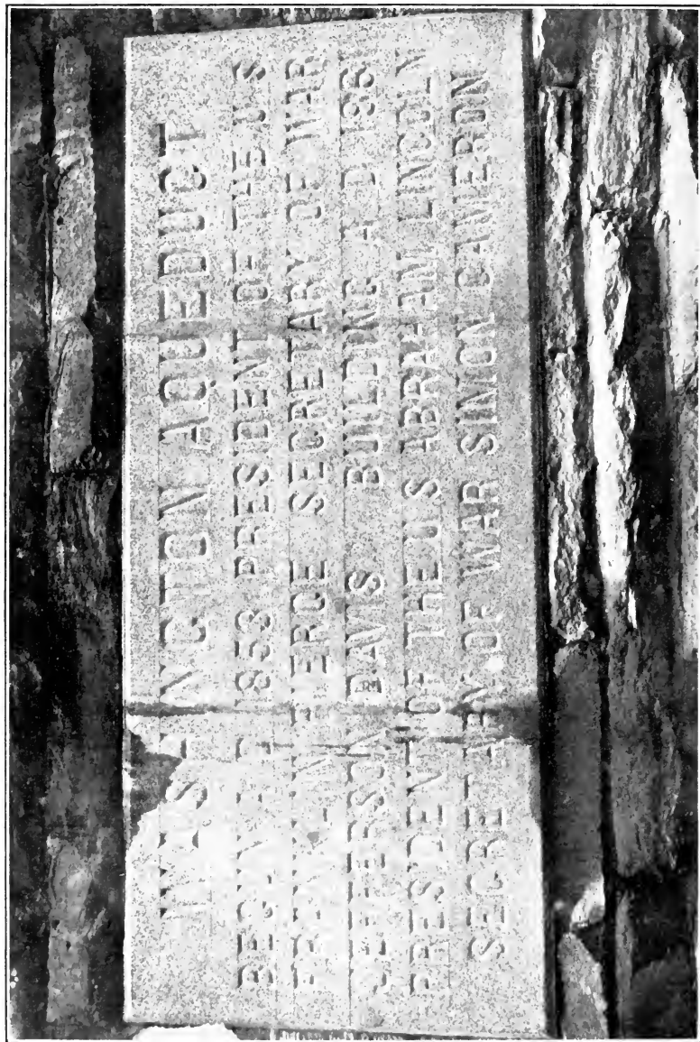
The entire tablet was "re-surfaced" without moving it from its position, and the original inscription, including the name of Jefferson Davis, was recovered.
