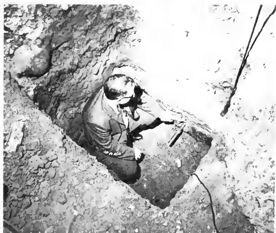
FIGURE 6. Engineer probings in basement of Ford's Theatre showing (left) blue clay foundations of north wall, and (right) rock and concrete foundations of south wall. The latter may be the original foundations of the First Baptist Church.
