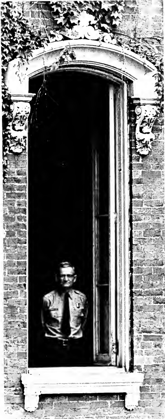
FIGURE 54. Detail of lintel and original casement window of south bay.
