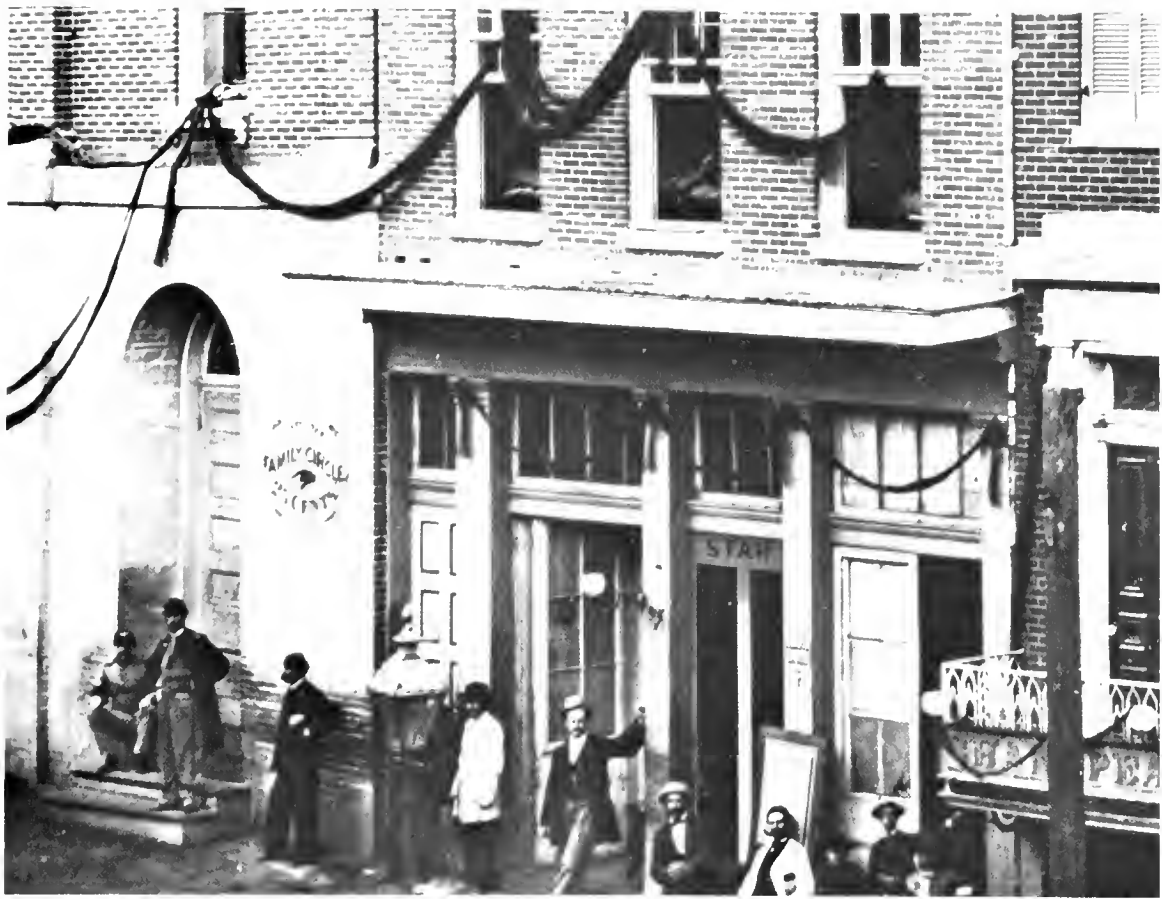
FIGURE 39. Closeup of façade of Star Saloon and possible location of theatre cornerstone.
