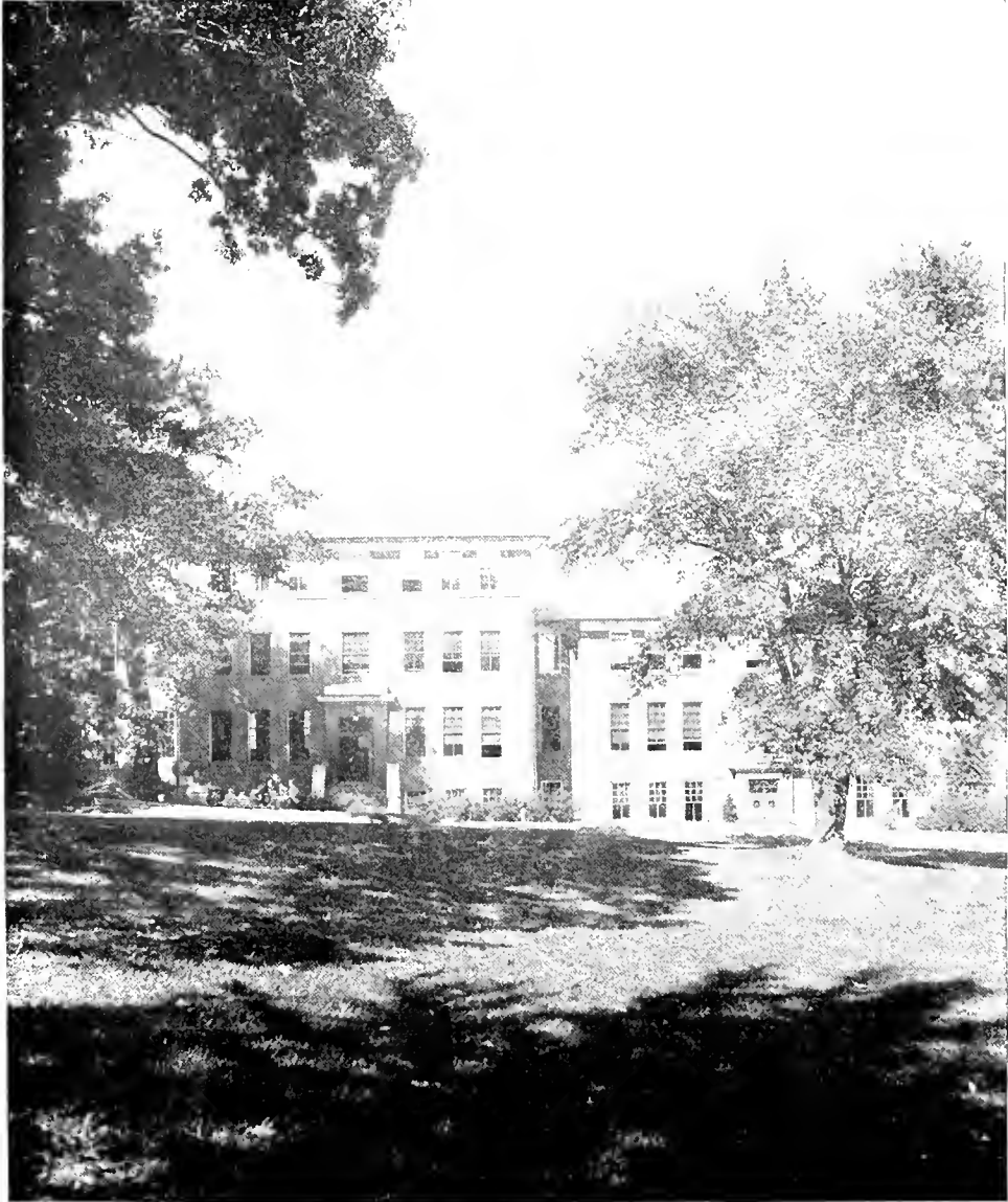
A PORTION OF THE ENGINEERING GROUP
