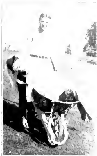
Wheeling it off after it was shoveled up
